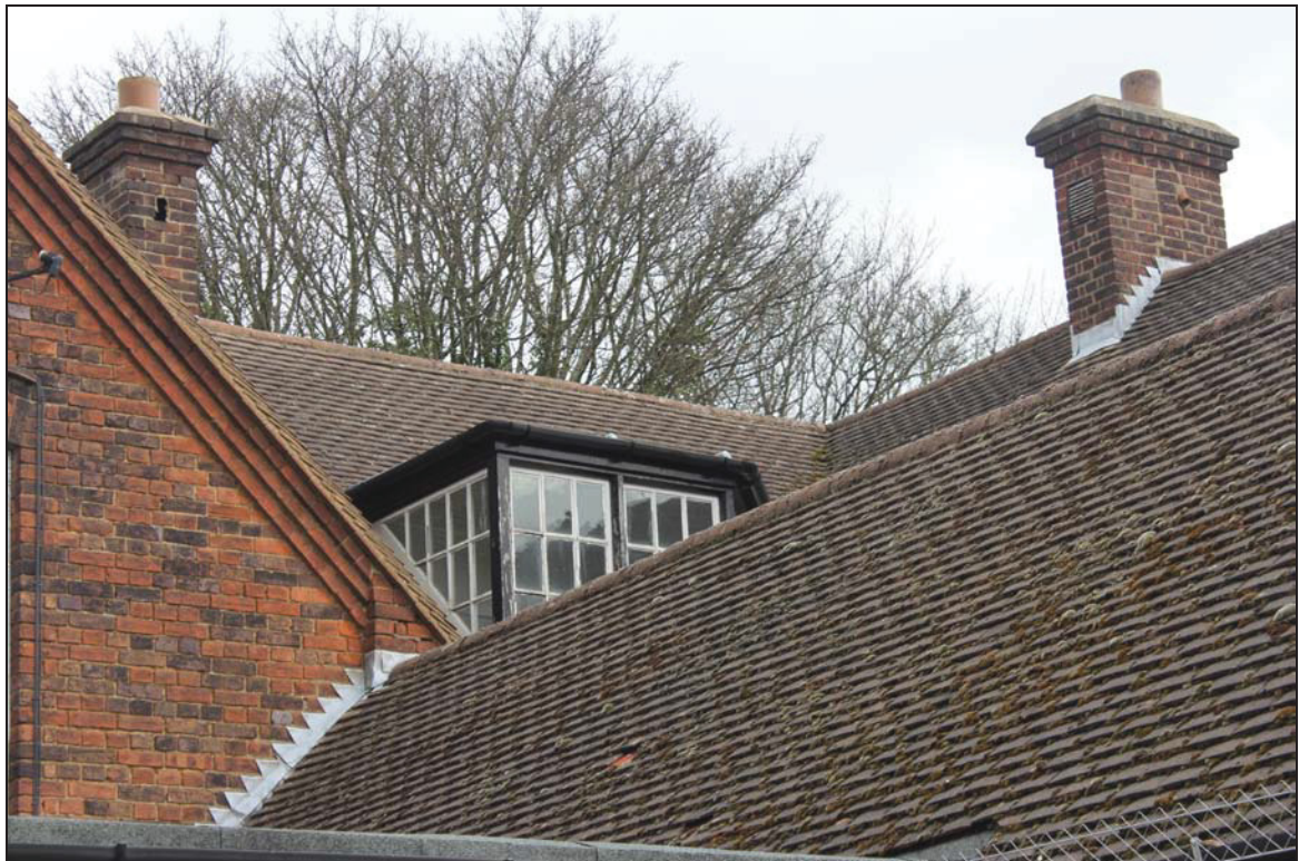
Plate 12 Dormer window on the south elevation, taken from the south (DP 09)
