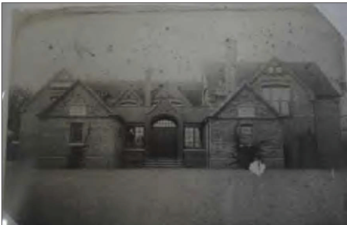
Photograph of the southern elevation of St Albans Board school, 1898 (HALS Ref: St Albans 515a-b)
