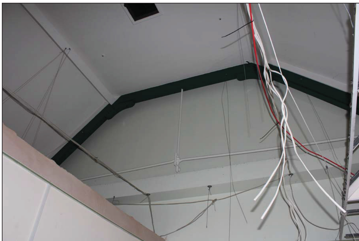
Plate 28 Roof structure in Classroom 3, taken from the north-west (DP 93)
