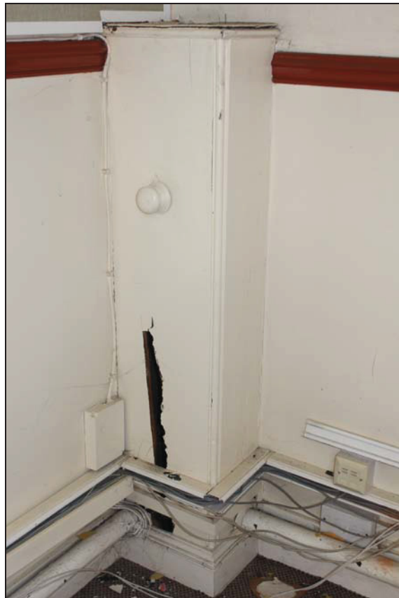
Plate 24 A thermostatic central heating unit in Classroom 2, taken from the south-west (DP 47)
