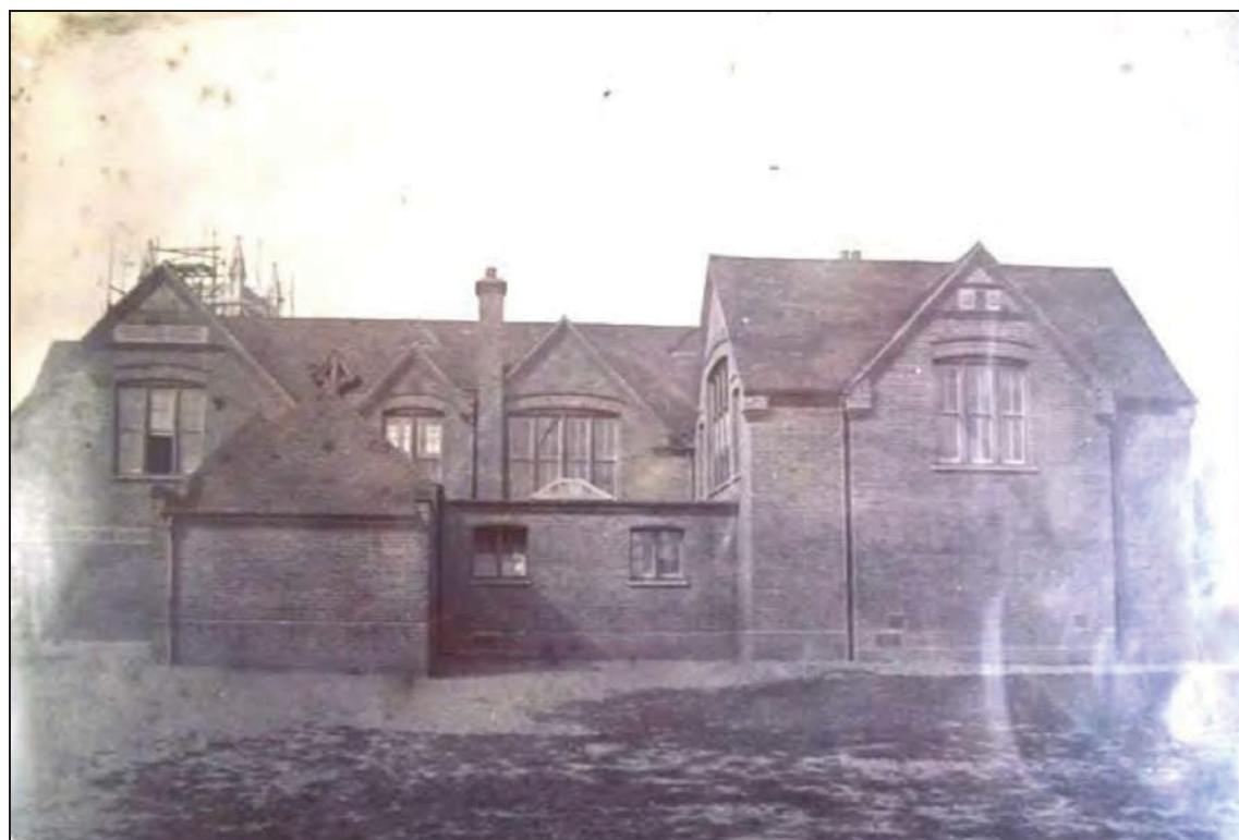
Photograph of St Albans Board School, viewed from the south c.1892 (HALS Ref: St Albans 505a-b)
