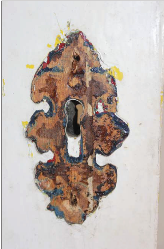
Plate 19 Evidence of historic paintwork under the key plate of the original external door of Classroom 2, taken from the east (DP 40)
