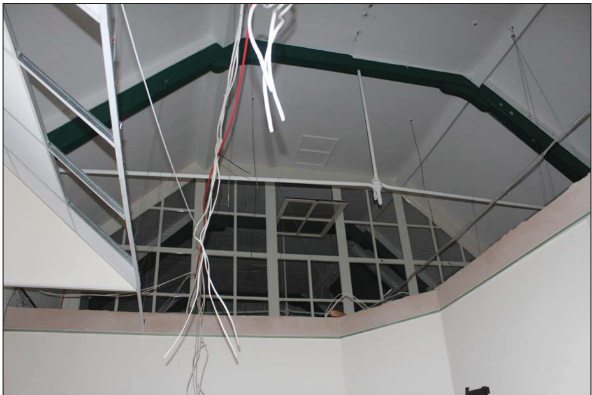
Plate 26 Glass partitions above Classroom 3, taken from the south (DP 26)
