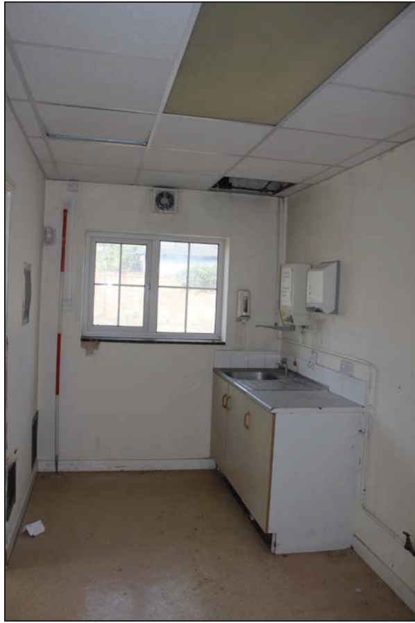
Plate 33 Kitchenette in the flat-roof extension, taken from the east (DP 75)
