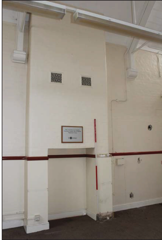
Plate 23 Chimney stack in Classroom 2, taken from the north (DP 43)
