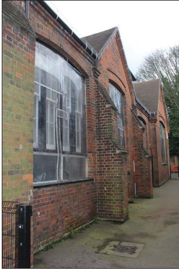
Plate 3 East elevation, taken from the south-east (DP 18)
