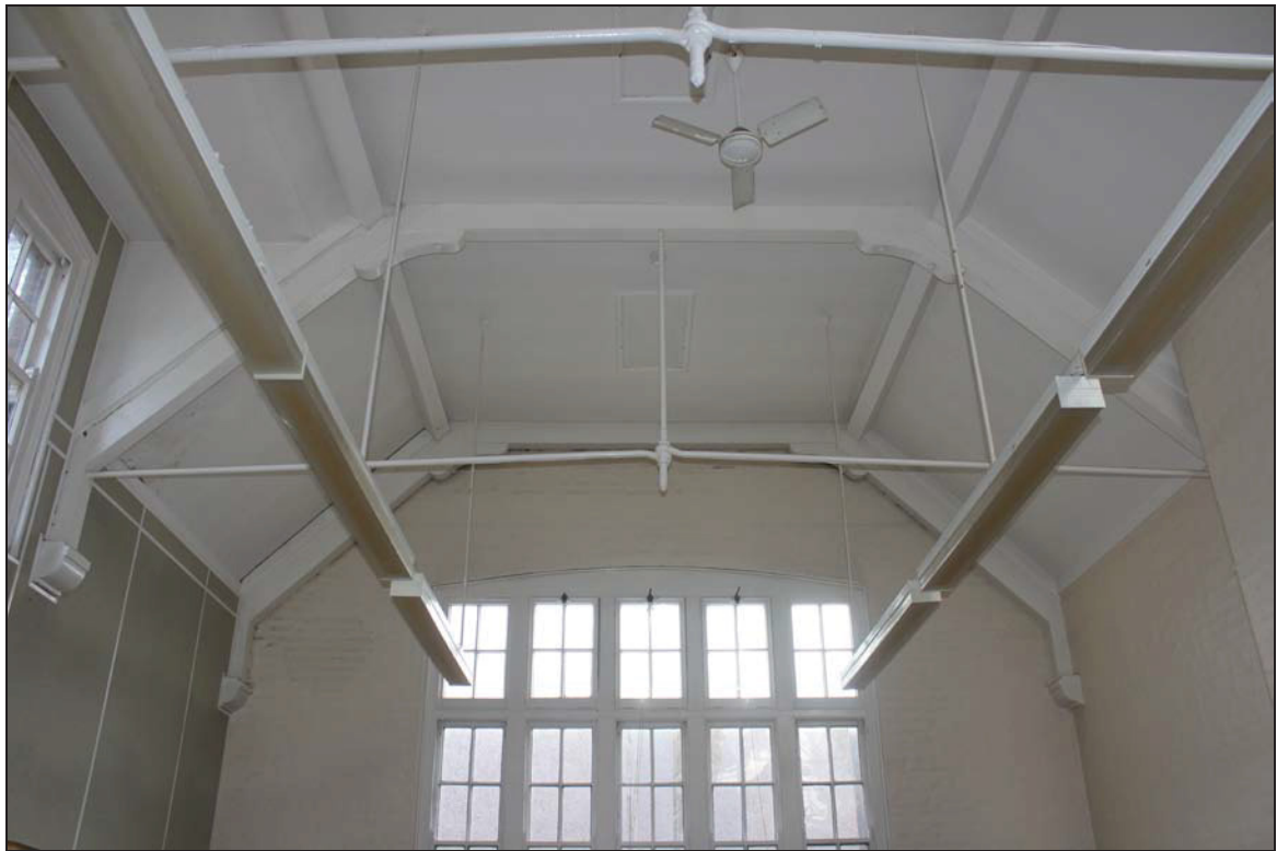
Plate 25 Roof structure in Classroom 2, taken from the west (DP 52)
