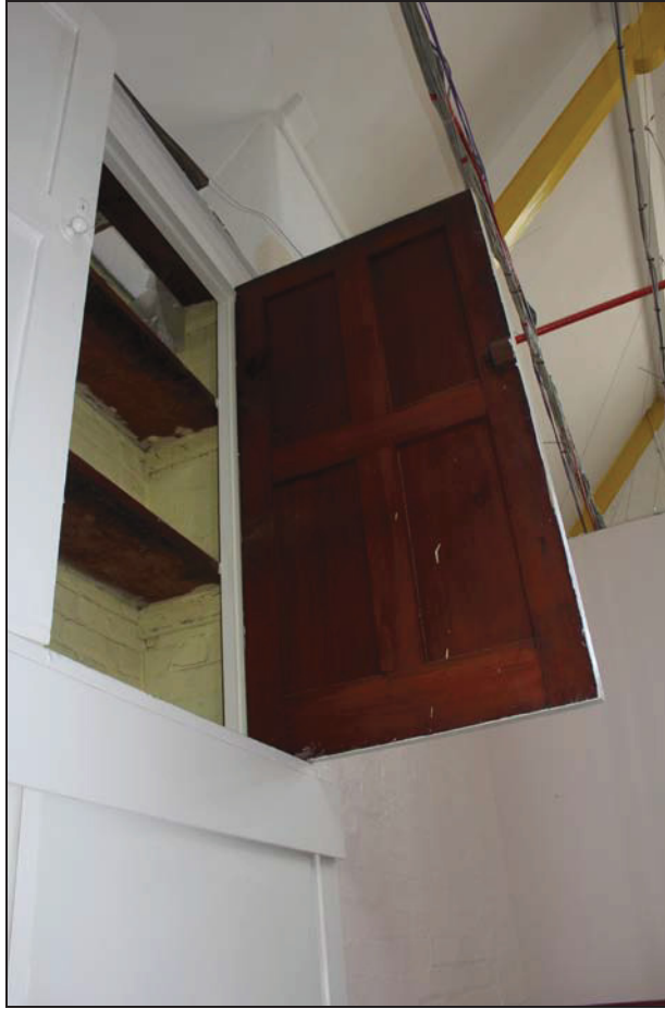
Plate 15 Internal cupboard door in Classroom 1, taken from the north (DP 32)
