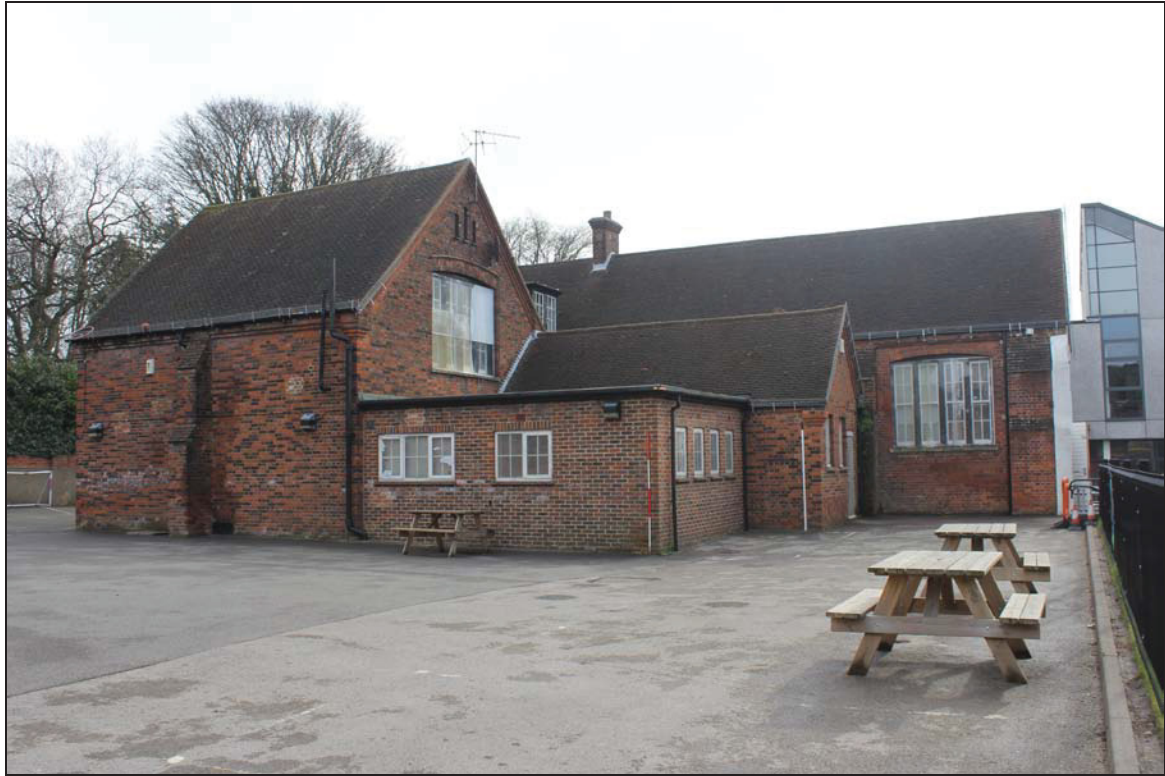
Plate 1 External view of the Pemberton Building, taken from the south-west (DP 01)
