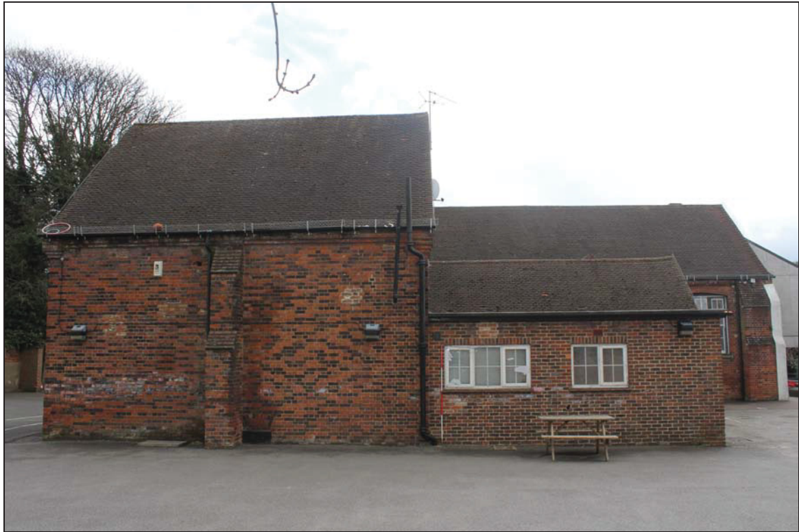
Plate 9 West elevation, taken from the west (DP 10)
