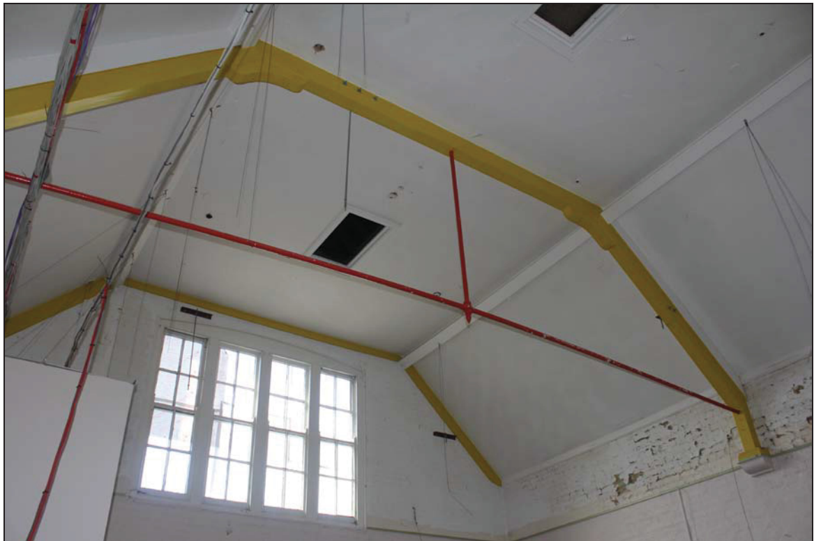
Plate 16 Roof structure in Classroom 1, taken from the north-east (DP 31)
