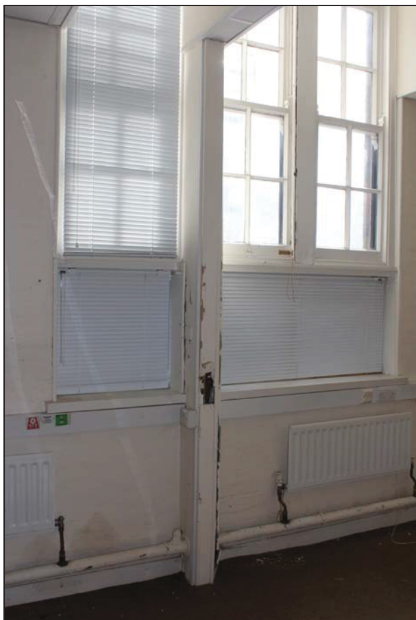
Plate 27 Provision for an internal partition in Classroom 3, taken from the north-west (DP 85)
