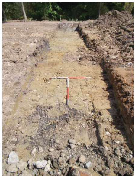
DP 12. Trench 3. Looking north-east.
