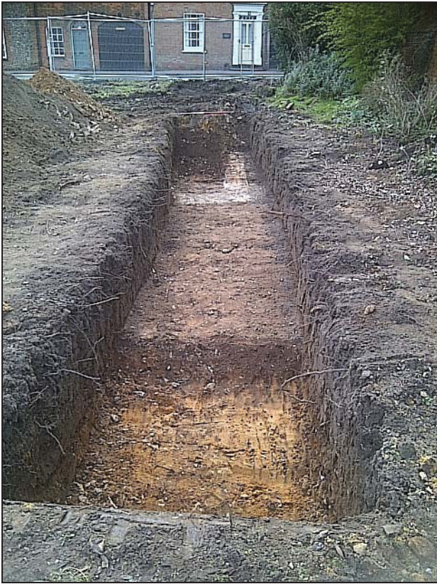
7 Post-excitation view of Trench 2 with test pits looking south-east
