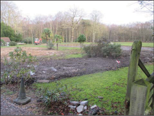
1 General view of site before excavating the trenches
