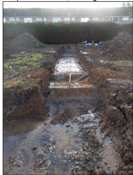
10 Trench 4 looking southwest.
