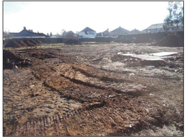
2 View of site looking south.
