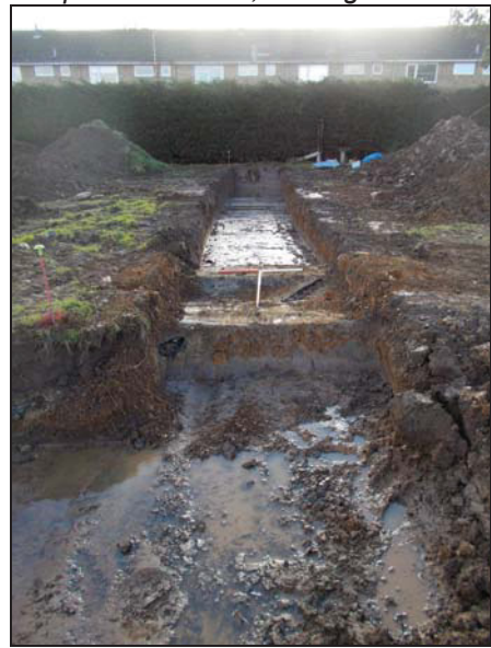
10 Trench 4 looking southwest.
