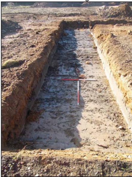
3 Trench 1 looking southwest.
