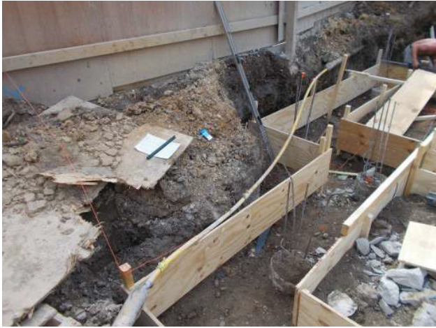
DP 7. South part of the site. Looking southwest.
