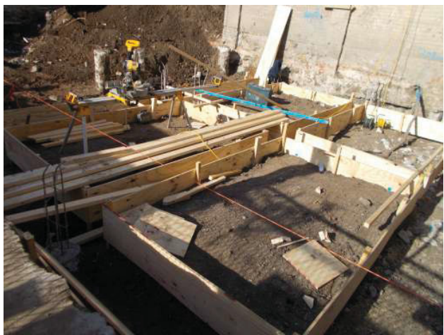
DP 5. Central part of the site. Looking south-west.
