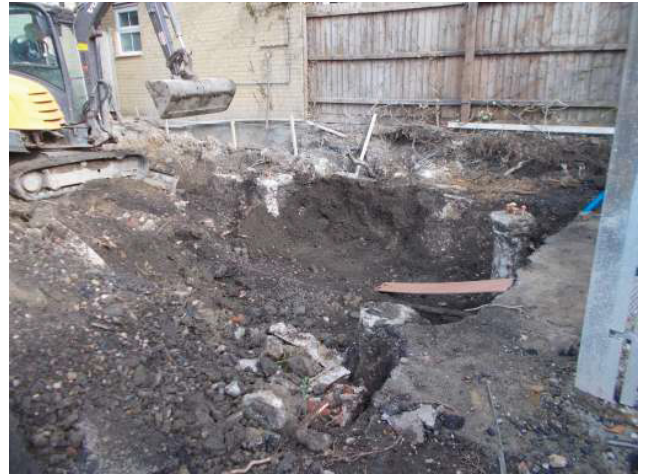
DP 2. Ground reduction in north part of the site. Looking north-west.
