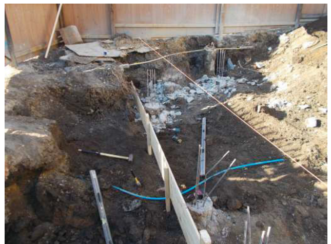
DP 6. South-east part of the site. Looking south.
