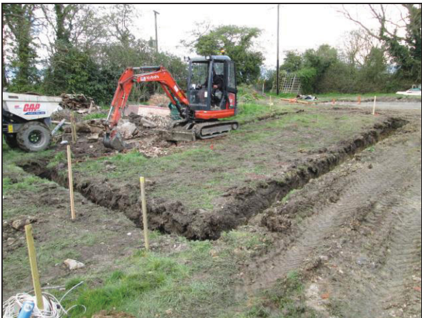
5 View of pool footings looking north
