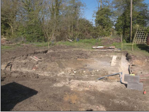
1 View of garden house footings looking north-west
