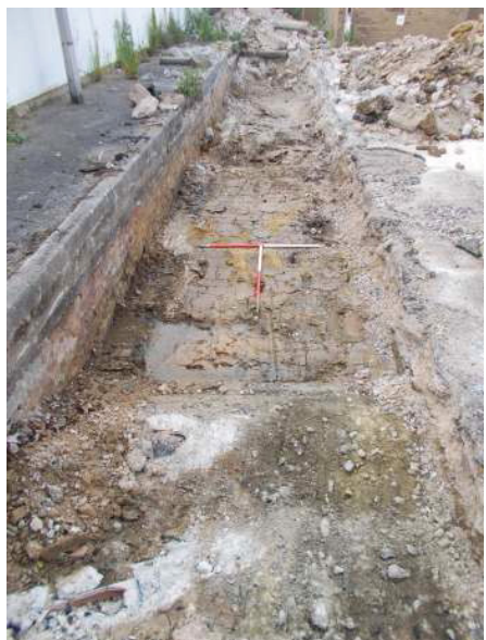
DP 6. Trench 3. Looking south.
