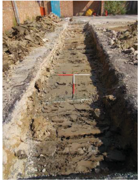
DP 2. Trench 1. Looking north.
