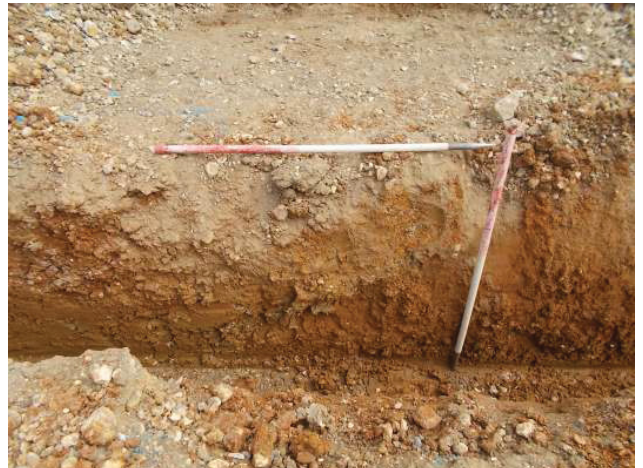
DP 4. East/central part of the site. Sample Section 2. Looking east-north-east.
