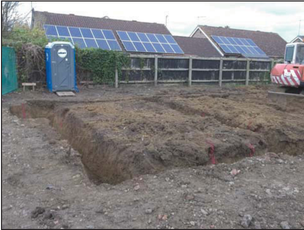
1 Post-excavation view of site looking north-east
