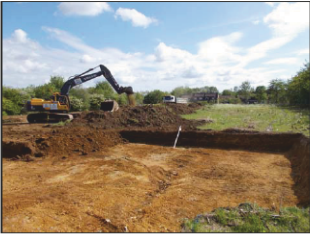
1 General shot of site during topsoil stripping
