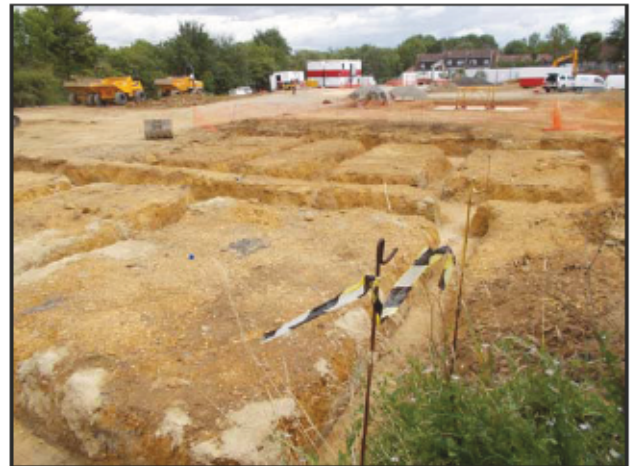
10 View of footings looking north-east
