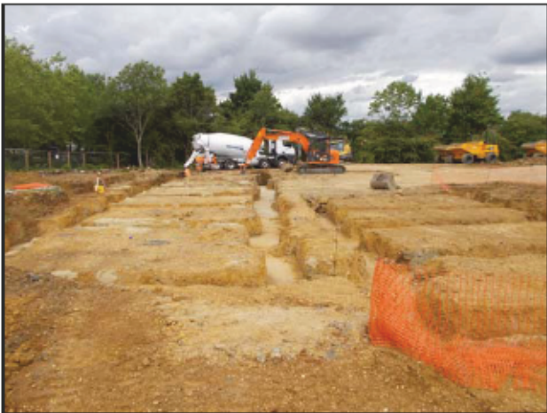
9 View of footings looking north
