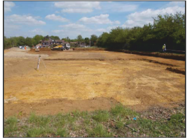
2 General shot of site after topsoil stripping
