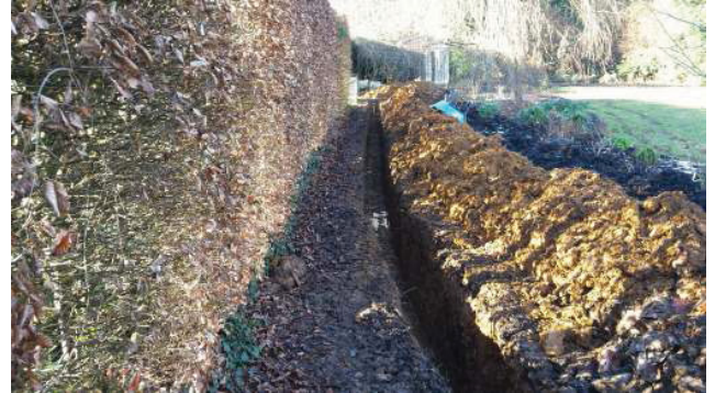
DP 8. Service trench with link to swimming pool. Looking south-west.
