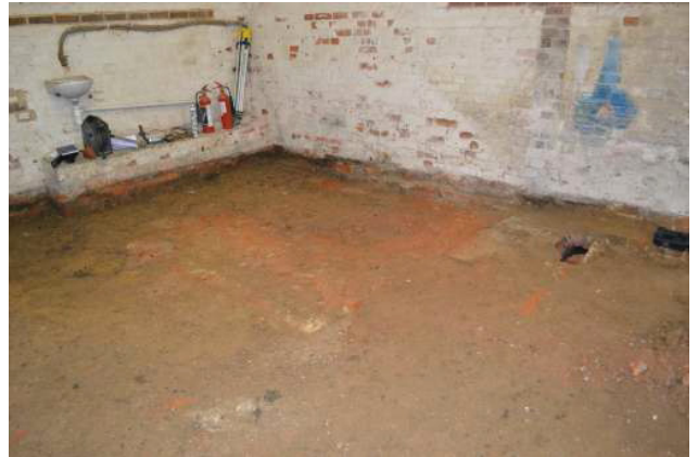
DP 2. Interior of the brewhouse. Looking east-south-east.
