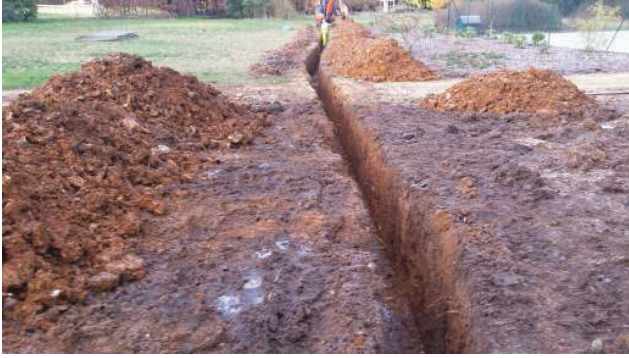
DP 7. Service trench with link to swimming pool. Looking west.
