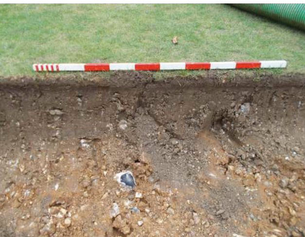
DP 5. Netball court. Sample section 3. Looking south-east.
