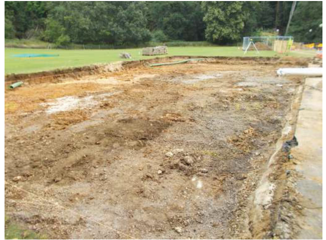
DP 2. North extension to netball court. Looking east.
