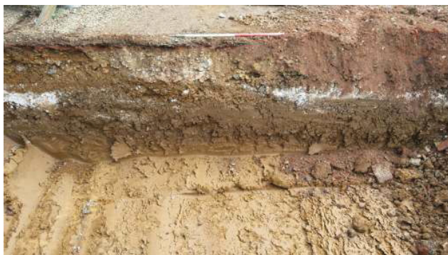
DP 17. Soakway Pit. Sample section 9. Looking east-south-east.
