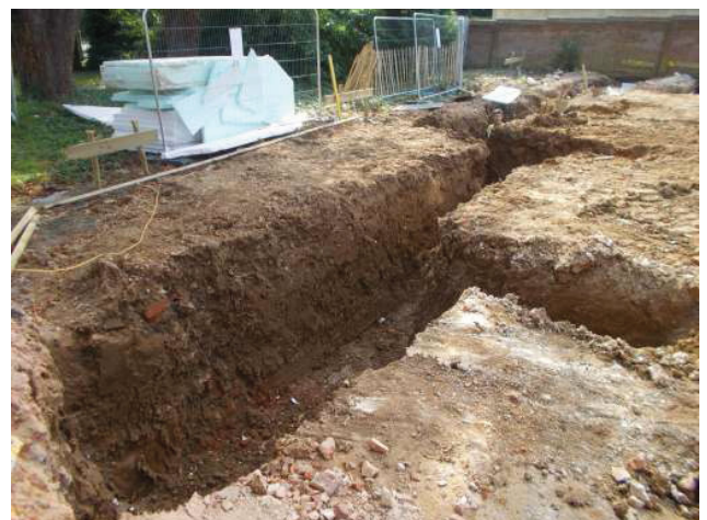
DP 12. Extension to Lodge Cottages. South foundation trench. Looking south-west.
