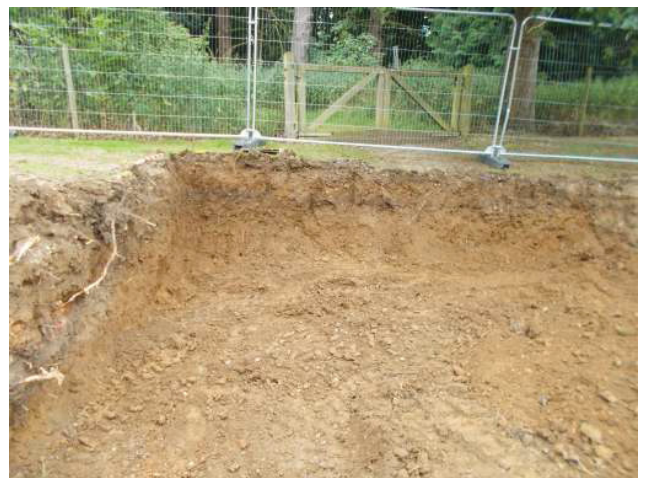
DP 6. Extension to car park. Looking north-east.
