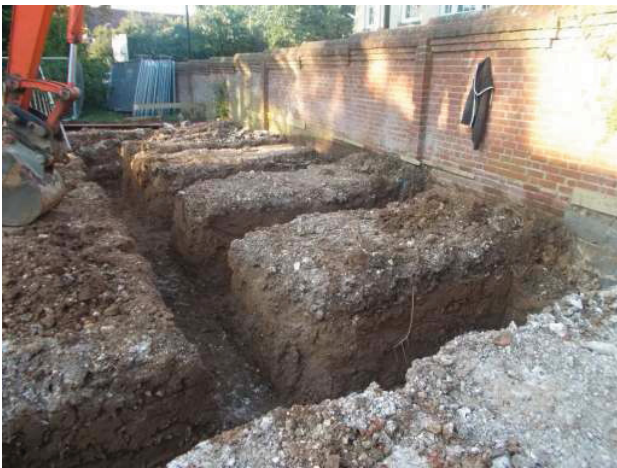
DP 9. Extension to Lodge Cottages. East foundation trenches. Looking south-south-west.
