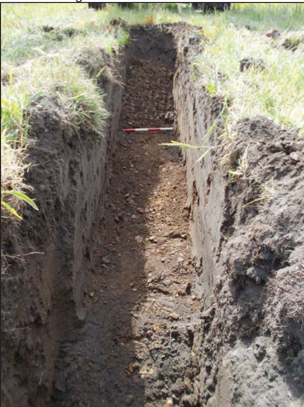
5 SW corner of foundation trench
