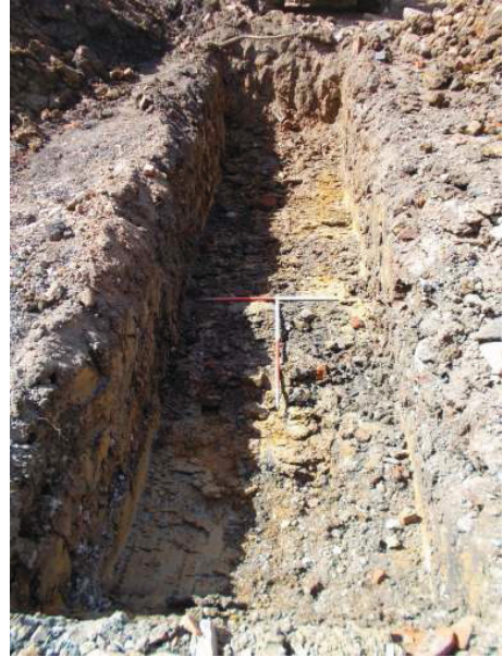
DP 8. Trench 2. Looking north-east.
