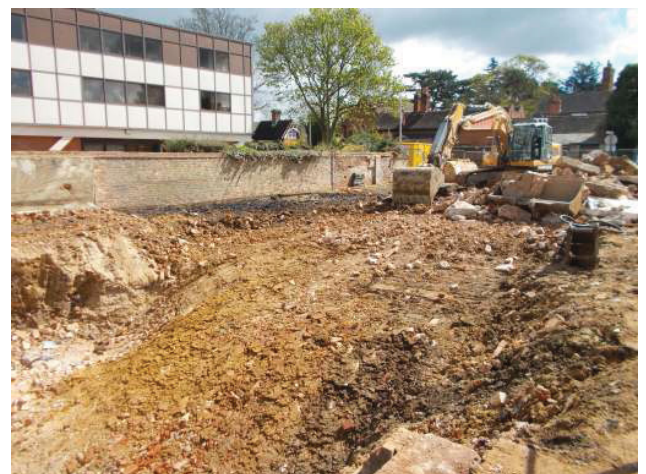
DP 12. Central part of the site during demolishing works. Looking south-east.
