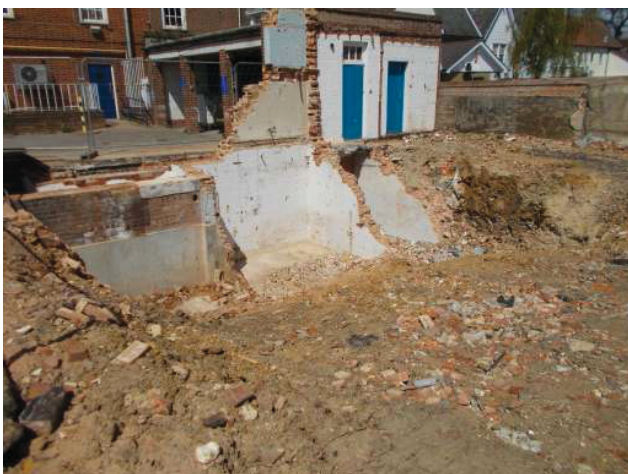
DP 11. North part of the site with basements exposed. Looking north-north-east.
