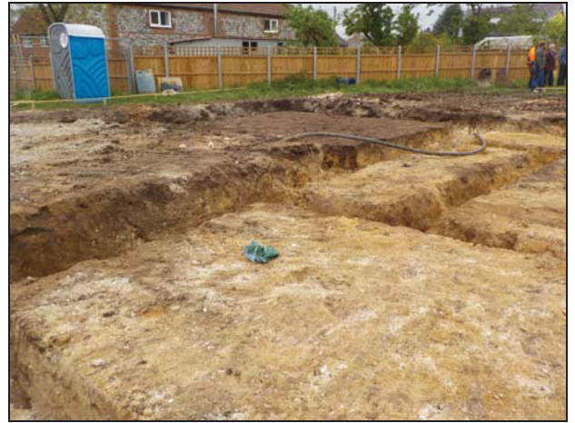
4 General view of site looking north-east
