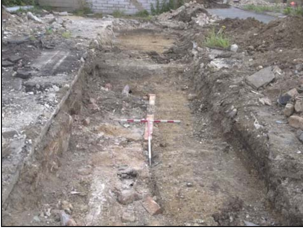
1 Post-excavation view of Trench 1 looking south-west
