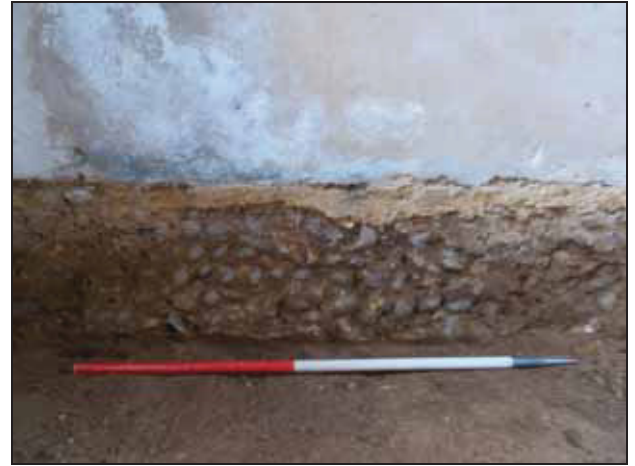
8 Wall M1001, looking east.
