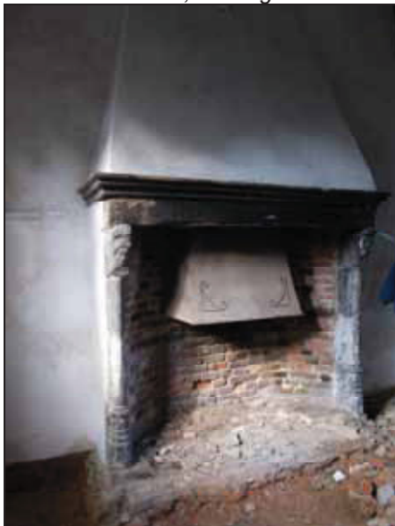
11 Fireplace at west end, looking west.
