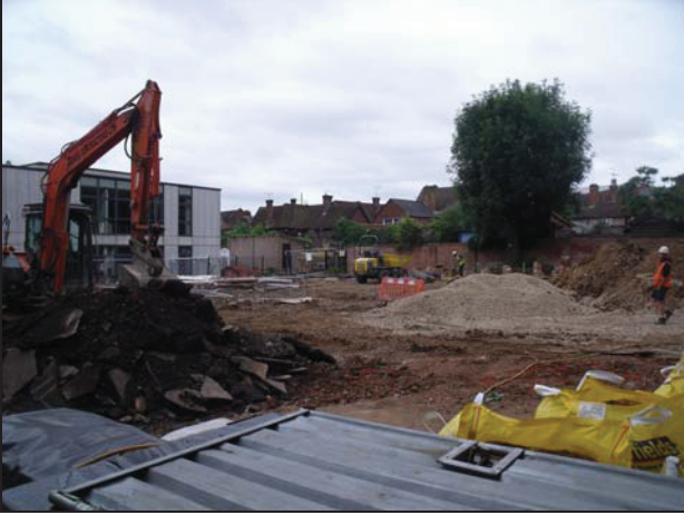
1 General view of site looking south-west
