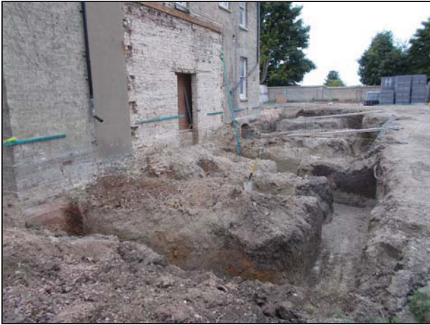
7 General view of site looking north-west
