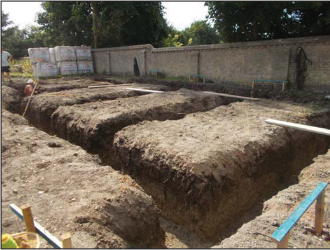
1 Garage block foundation trenches. Looking west
