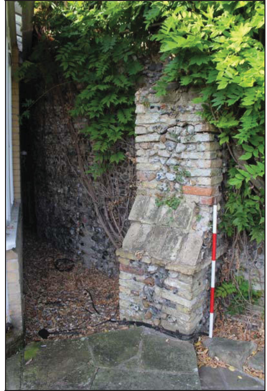
15 Buttress on the east side of the curved wall, looking north-west
