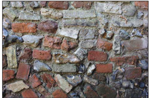
21 Sample of brick and flint on the north-west side of the curved wall showing brick of varying dates, looking south-east
