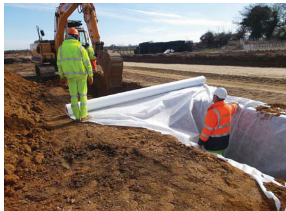
12: Backfilling of soakaway trench across Clay Lane, looking NW
