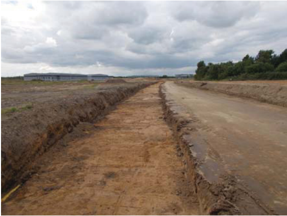
13: Subsoil strip between Roundabout D and Excalibur Road, looking SE
