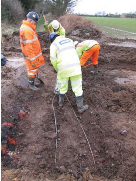
3: Removal of telecommunications cable (Clay Lane), looking S
