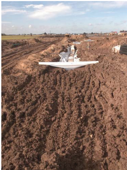
9: Backfilling of soakaway trench between Roundabouts A and B, looking W
