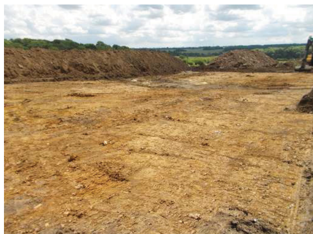
DP 2. The site. Looking south-east.
