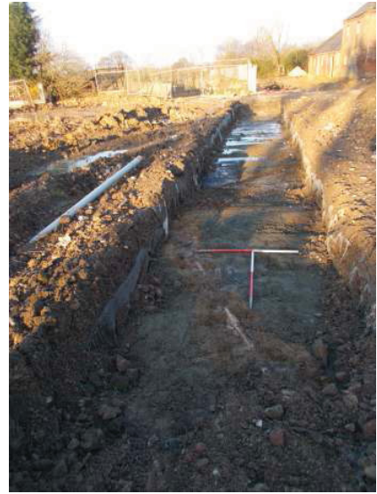
DP 2. Trench 1. Looking north-north-east.
