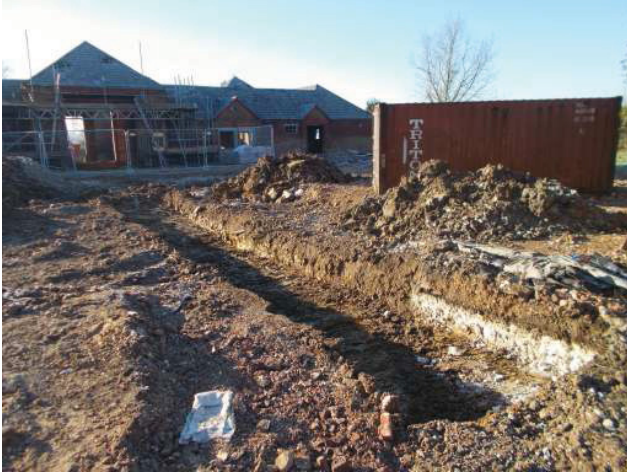
DP 13. Trench 4. Looking south-west.
