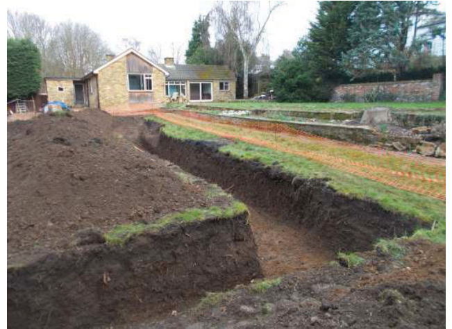
DP 8. Trench 3. Looking north-east.
