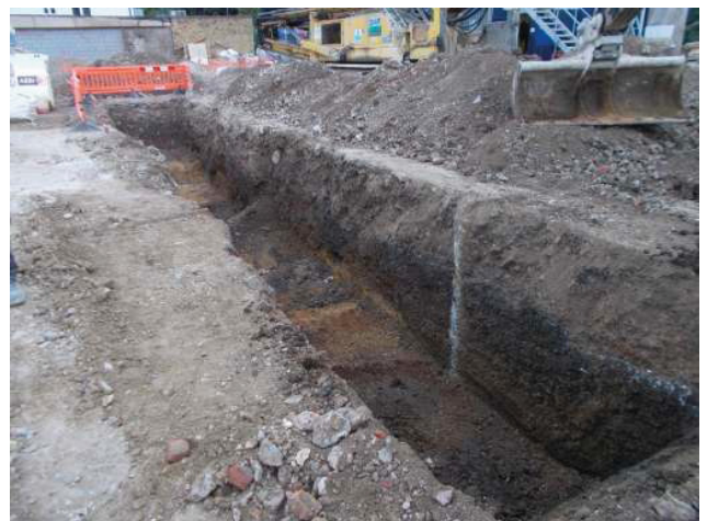
DP 6. Trench 2. Looking east-north-east.
