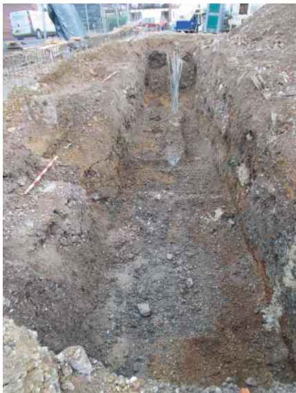
DP 3. Trench 1. Looking west-north-west.
