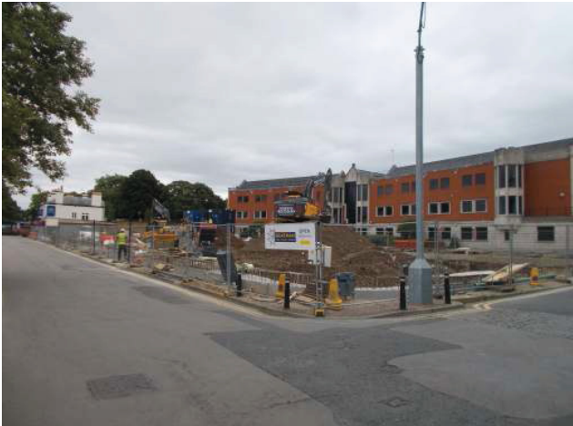
DP 1. The site. Looking east.
