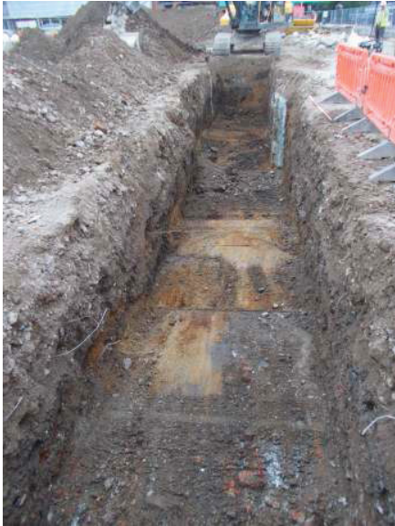
DP 7. Trench 2. Looking south-west.
