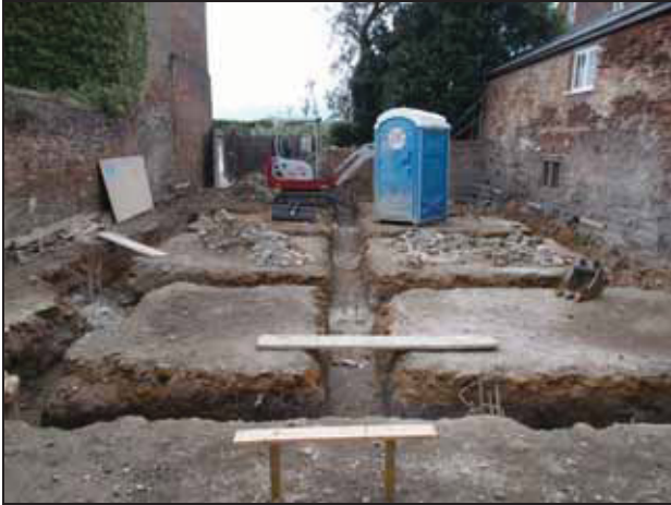
1 General shot of site after excavation of footings
