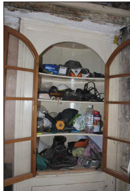
DP 24 Detail of the cupboard showing shaped display shelves (GF01; main range), taken from the north-west
