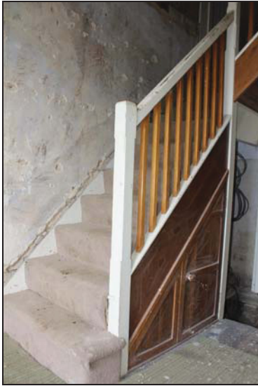
DP 19 Staircase in entrance vestibule GF02, taken from the west
