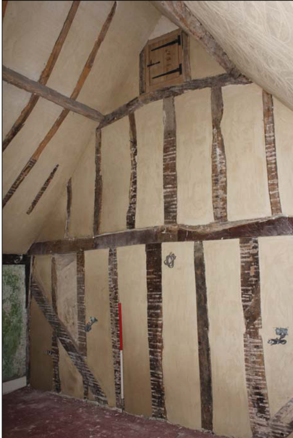
Plate 10 Timber-framing on the south-west wall of Room FF01 (main range), taken from the north (DP 54)
