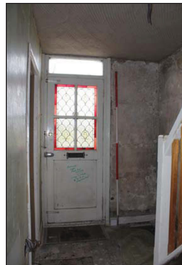
DP 18 Entrance/stair vestibule GF02, taken from the south-east
