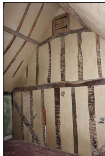
Detail of the south-east wall of Room FF02 (Unit 2) showing now truncated wall-plate of the historic core with tie-beam end above, taken from the north-west
