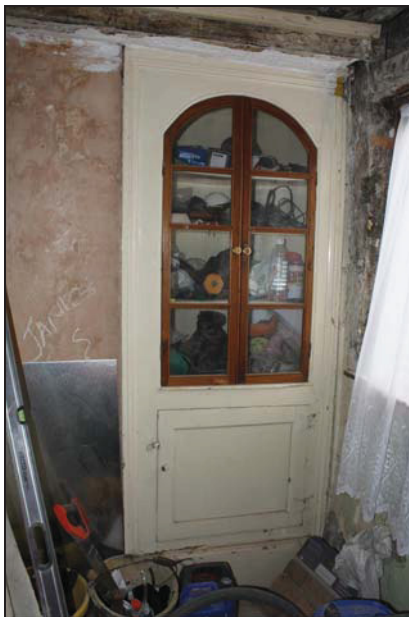
DP 23 Early 18 th century fitted cupboard in the south corner of Room GF01 (main range), taken from the north-west
