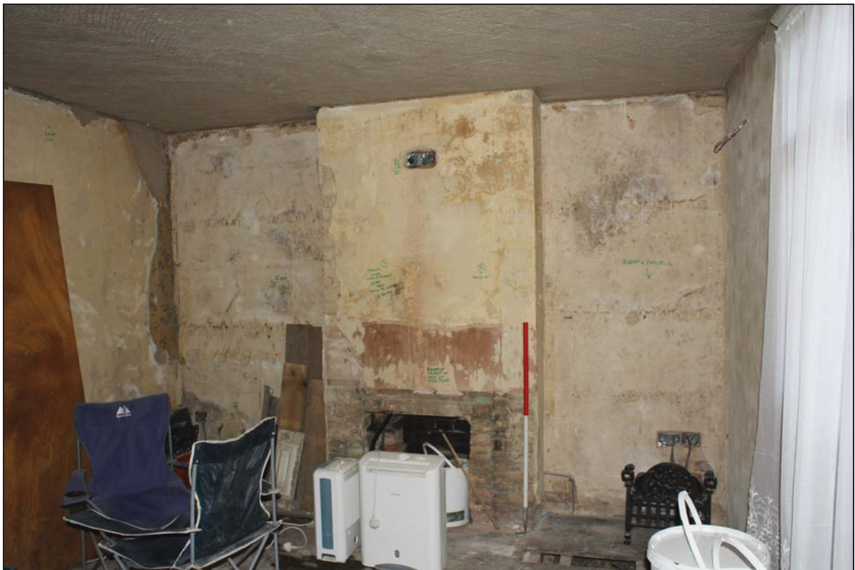
Plate 9 South-west side of Room GF03 (Unit 2), taken from the north-east (DP 8)
