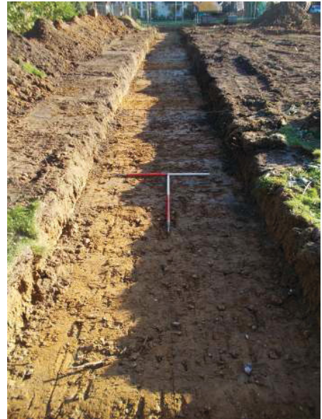
DP 10. Trench 3. Looking south-south-east.
