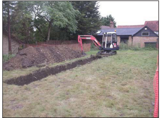
4 View of site looking north-west
