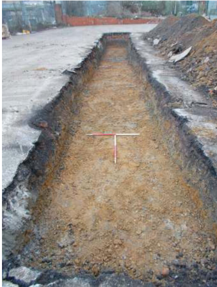
DP 7. Trench 2. Looking north-east.
