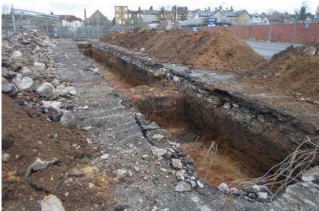
DP 11. Trench 3. Looking north-north-west.
