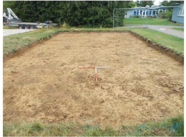
DP 2. Area of investigation. Looking north-north-west.
