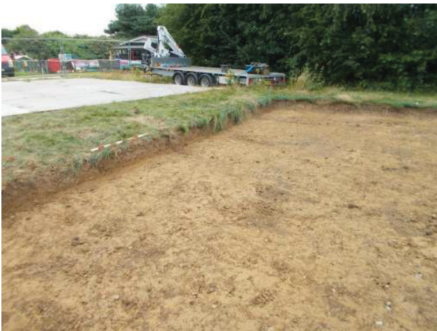
DP 5. West part of the area with sample section 2. Looking north-west.
