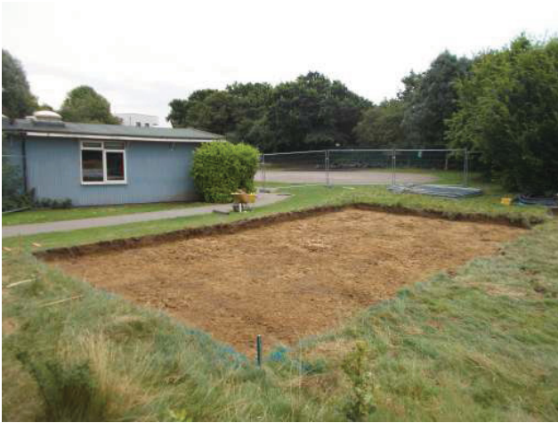
DP 1. Area of investigation. Looking south-east.
