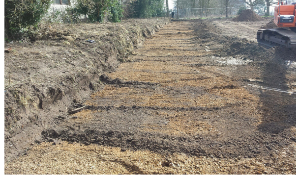
DP 2. Stripping along northern edge of site. View south-east.
