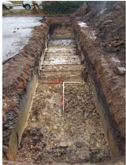
DP 4. Trench 1. Looking south-south-west.
