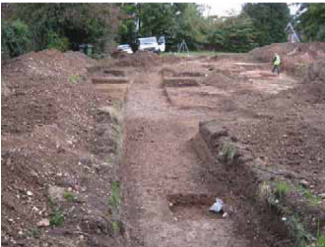
DP 3. The north-west part of the site. Looking south-east.
