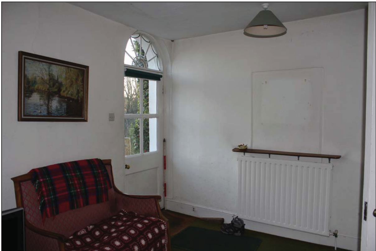
Plate 12 West side of Room GF04 showing reeded surround outlining the position of an original doorway, taken from the north-east (DP 47)
