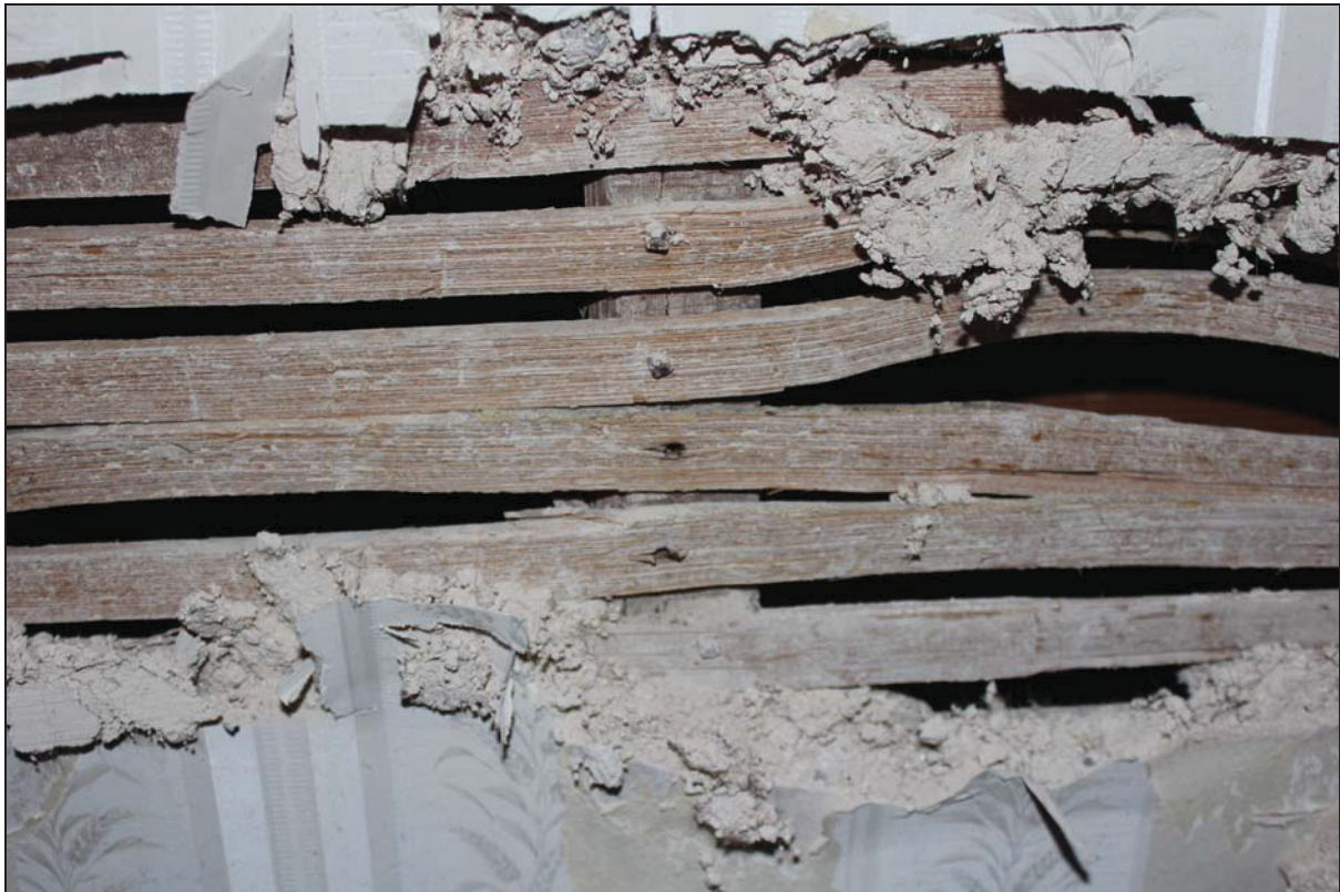
Plate 14 Detail showing the nailed laths in the small intervention on the west side of Room FF01, taken from the east (DP 75)
