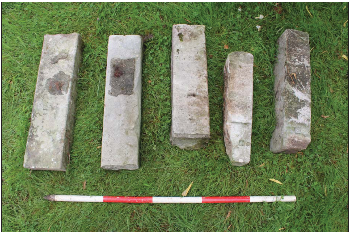
Plate 6 Number of fragments of the probable original external steps reused in later landscaping (DP 116)
