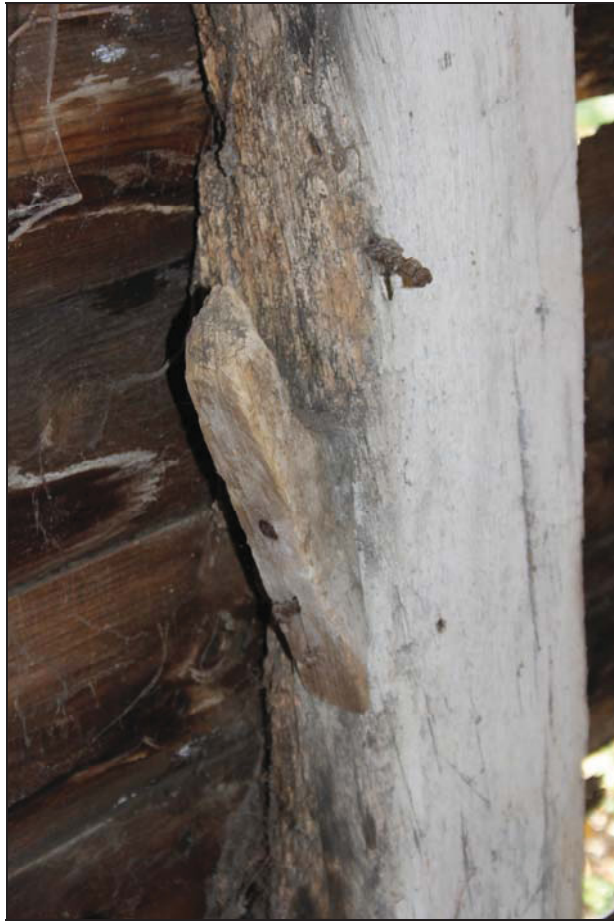
Plate 27 Wooden hook within the outshut of Building 2, taken from the east (DP 76)
