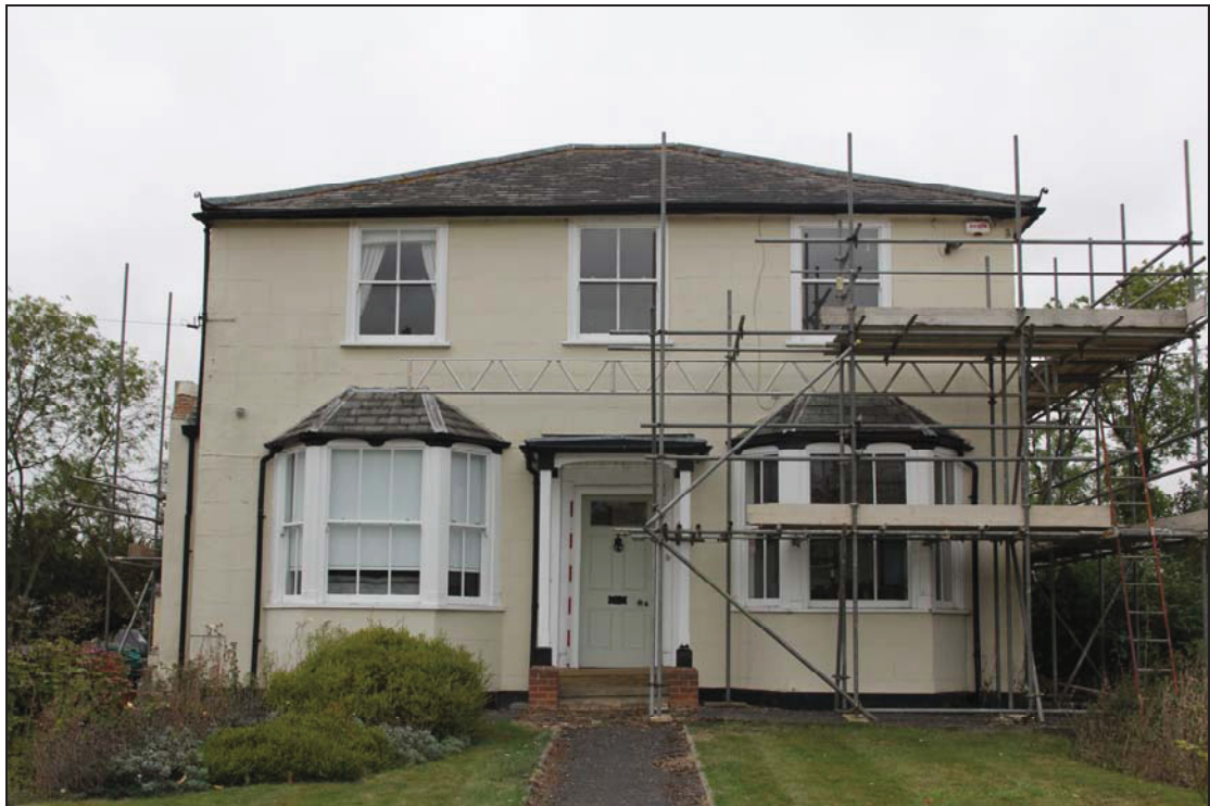
Plate 1 Front elevation of Building 1, taken from the south-east (DP 01)
