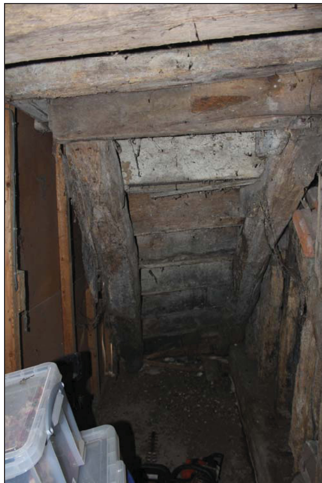
Plate 18 Carcass of the staircase in Building 2, taken from the north-west (DP 64)
