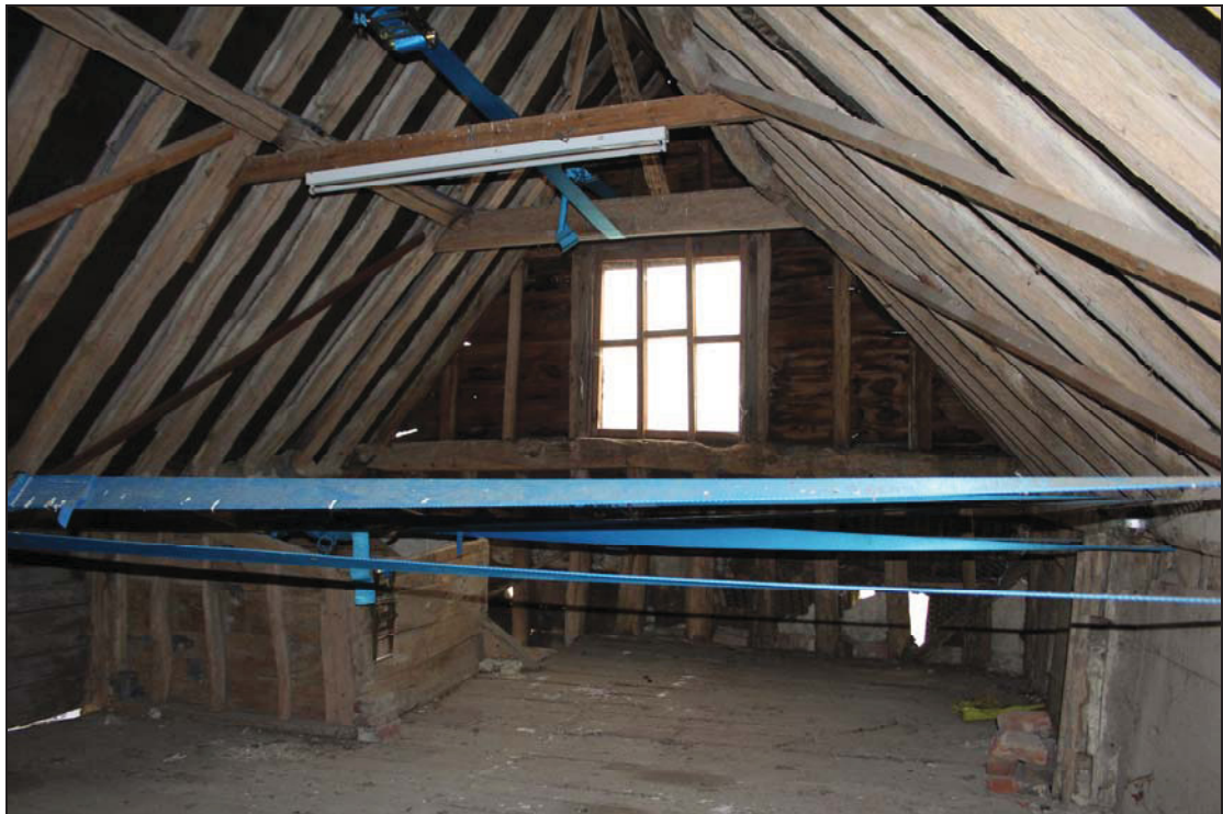
Plate 22 First floor of Building 2, taken from the north (DP 49)
