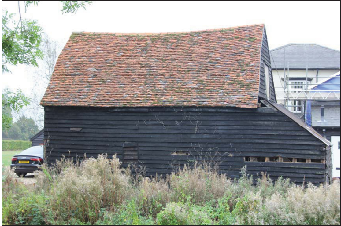
Plate 11 Side elevation of Building 2, taken from the north-west (DP 15)
