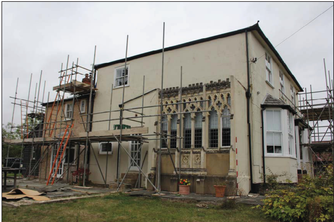
Plate 2 Side elevation of Building 1, taken from the south (DP 05)
