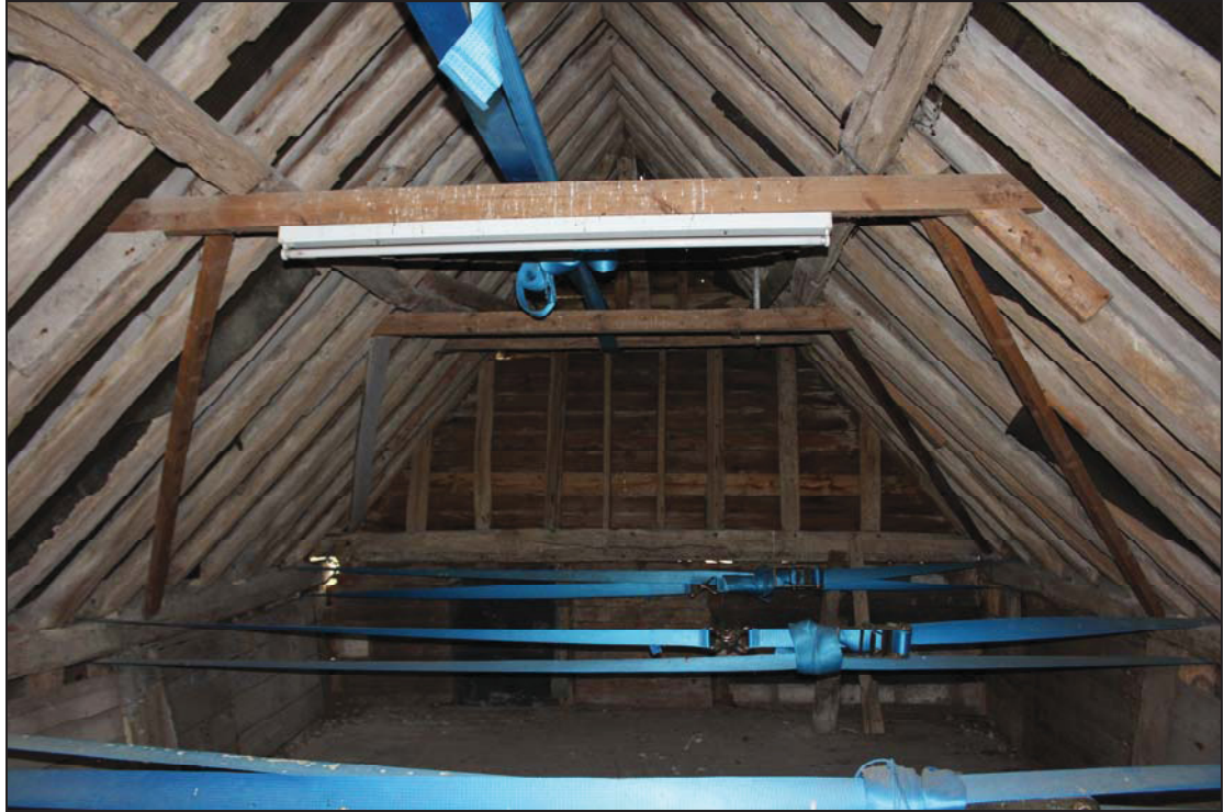
Plate 23 First floor of Building 2, taken from the south-west (DP 46)
