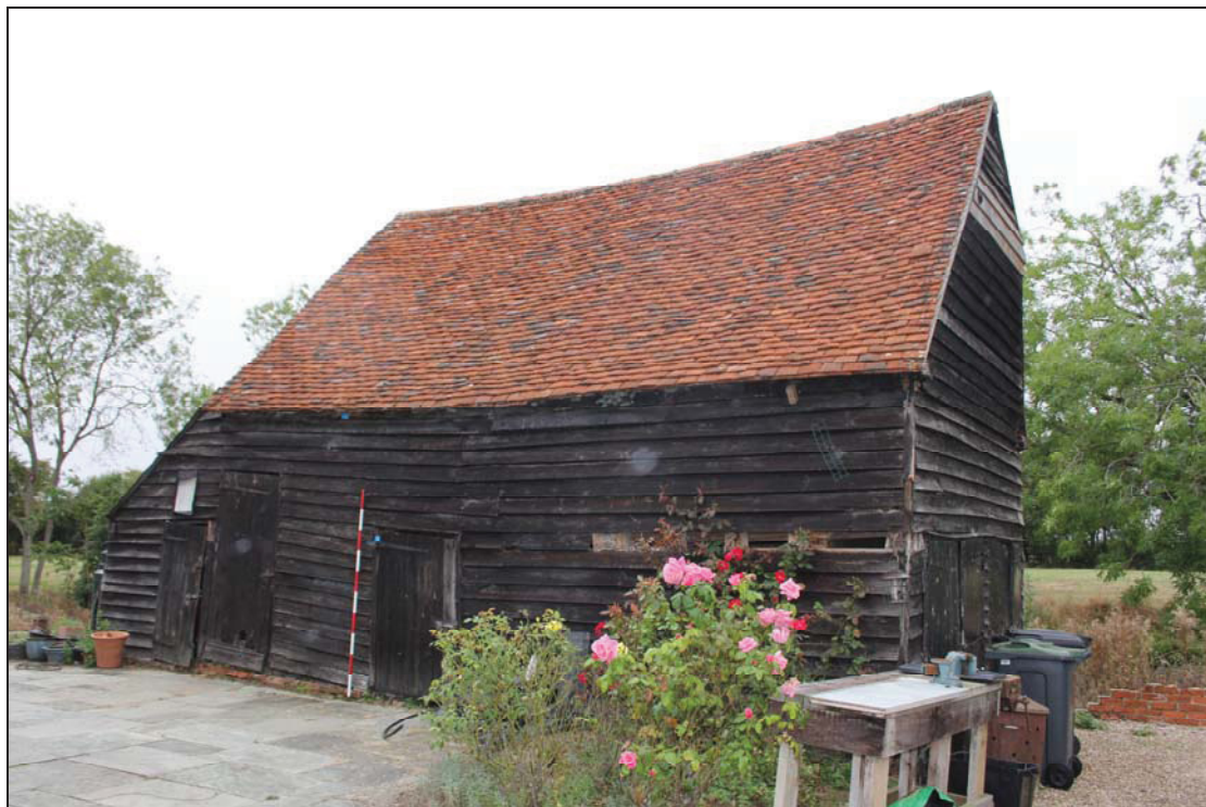
Plate 10 Exterior of Building 2, taken from the east (DP 11)
