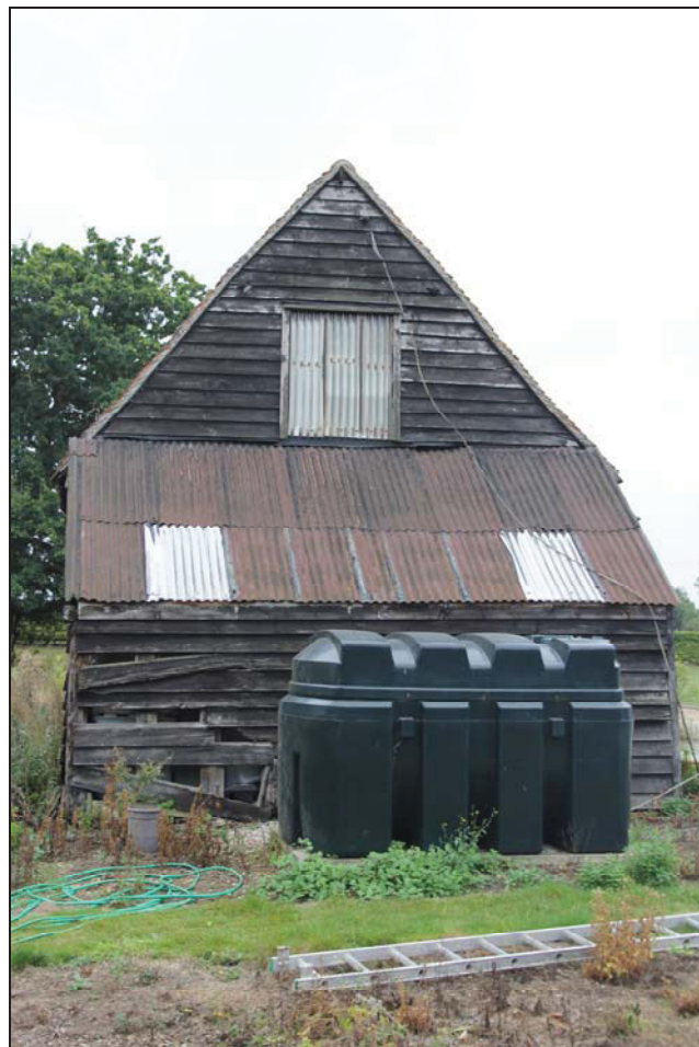
Plate 12 Gable end of Building 2, taken from the south-west (DP 13)
