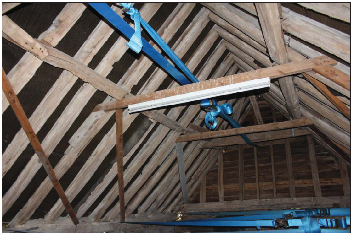
Plate 24 Roof structure in Building 2, taken from the south (DP 53)
