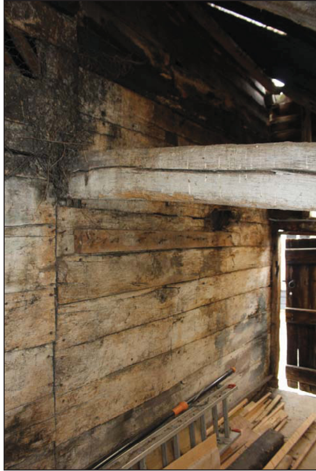
Plate 25 Weather-boarding along the original external wall of the main barn in Building 2, taken from the west (DP 59)
