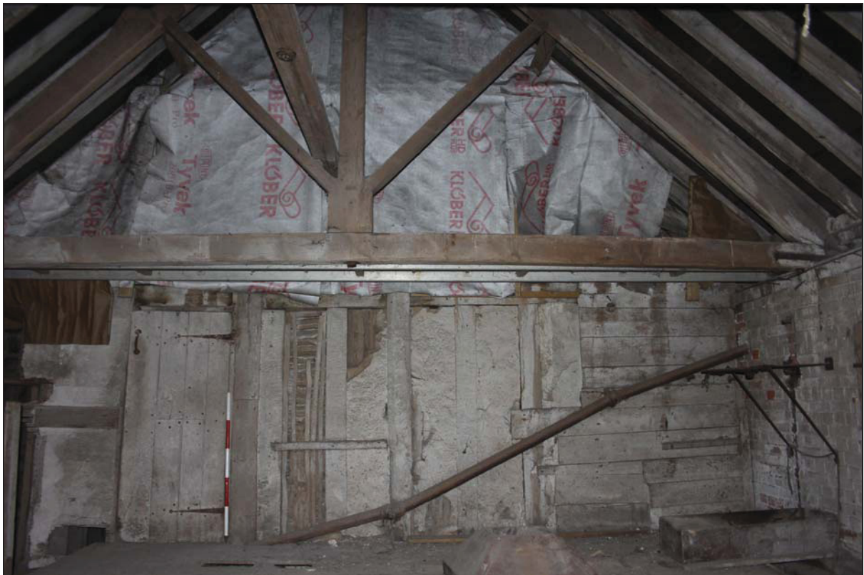
Plate 10 Part of the original exterior south elevation of the tithe barn, previously protected by a precursor (DP 30)
