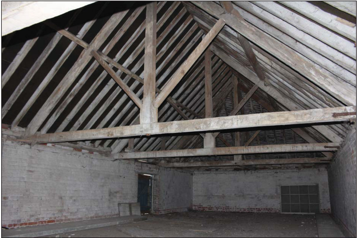
Plate 9 Roof structure of Building 1, taken from the south-east (DP 31)
