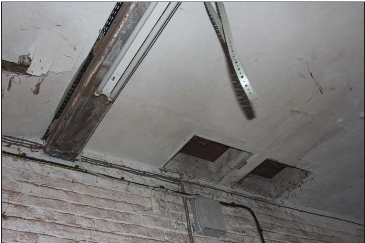
Plate 6 Hatches for dropping hay from the first floor in Building 1, taken from the east (DP 05)
