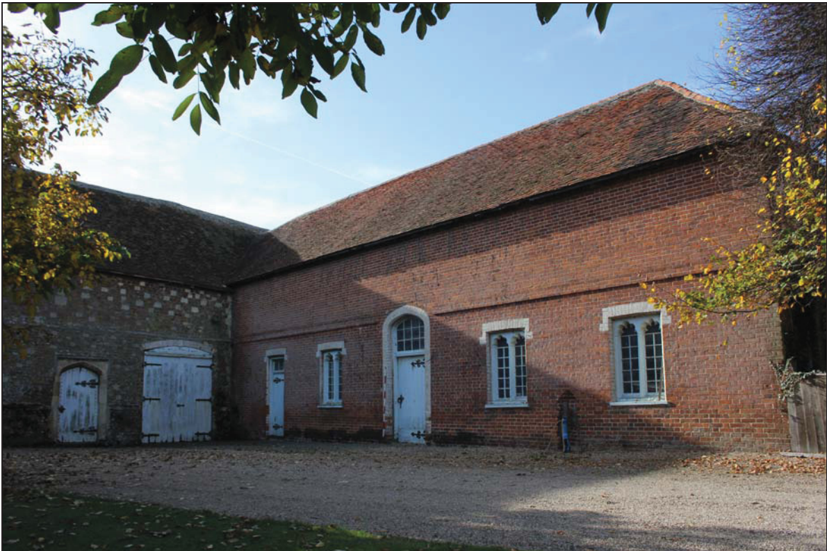
Plate 1 East elevation of Building 1, taken from the north-east (DP 58)
