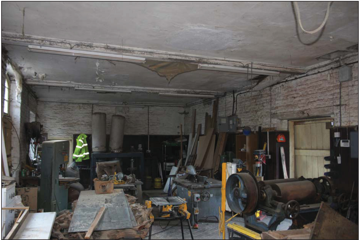
Plate 5 Interior of Building 1, taken from the north (DP 02)
