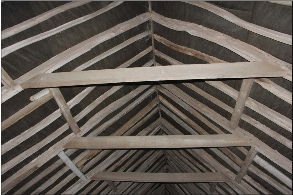
Plate 13 Roof structure in Building 2, taken from the north (DP 77)
