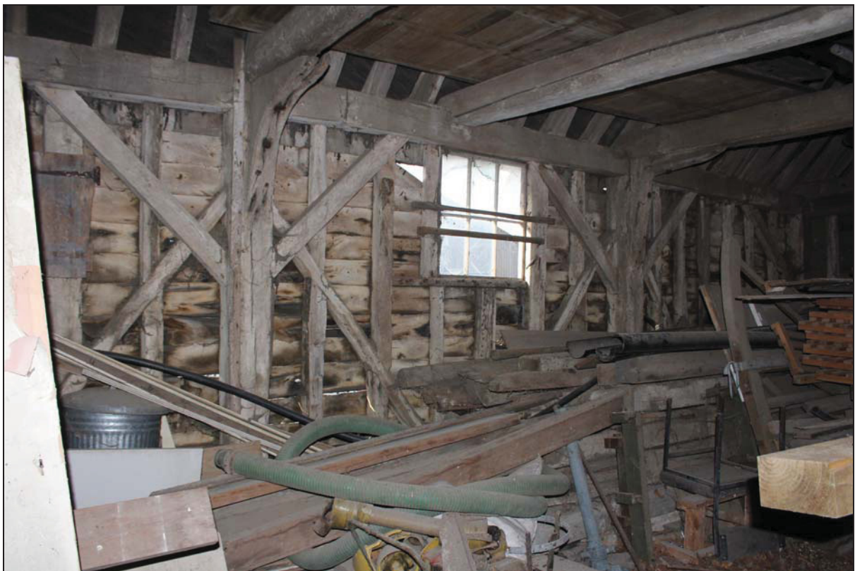
Plate 14 West side of Bay 3 in Building 2, taken from the south-east (DP 86)
