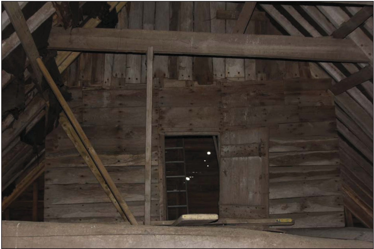
Plate 15 Loft above Bay 6 in Building 2, taken from the north (DP 91)
