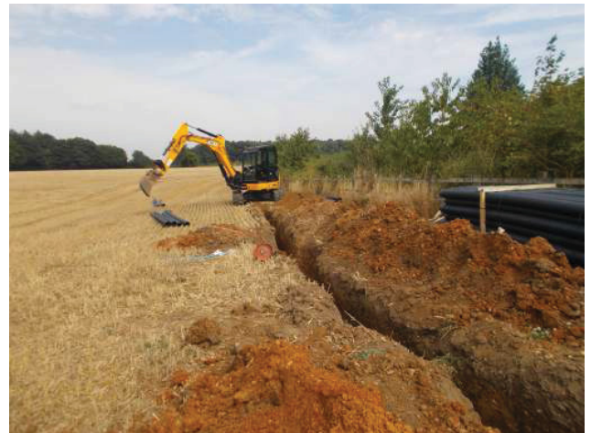
DP 10. Field north-west of the village. Cable trench, looking north.
