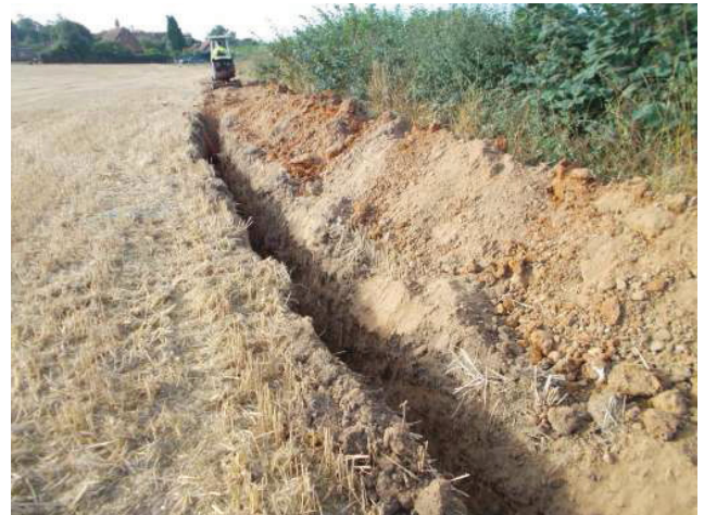
DP 4. Field north of the village. Cable trench, looking south.
