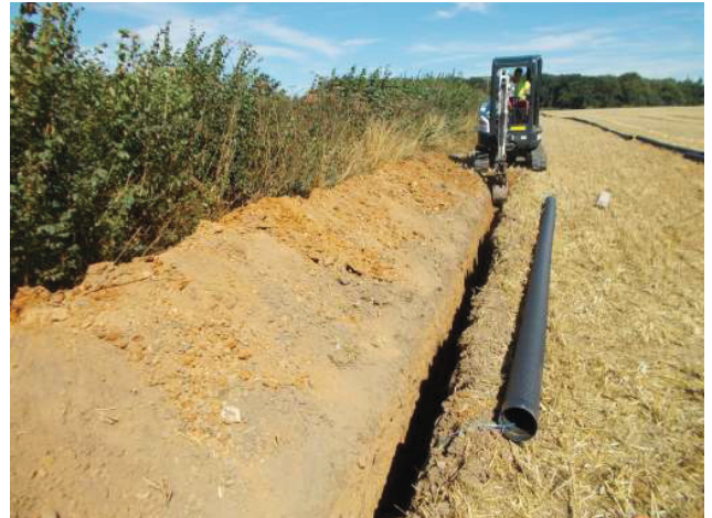
DP 2. Field north of the village. Cable trench, looking north-north-west.
