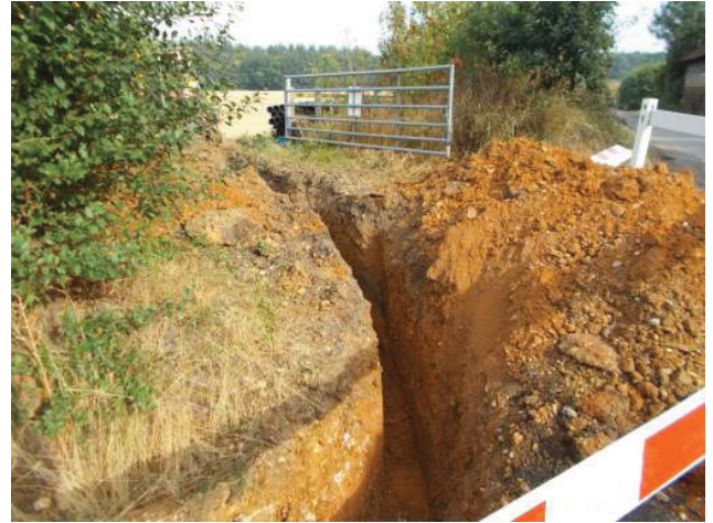
DP 8. Access to field north-west of the village. Looking north-west.
