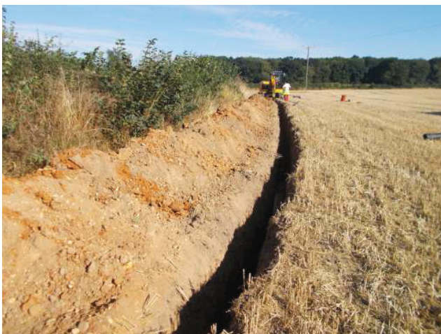
DP 5. Field north of the village. Cable trench, looking north.
