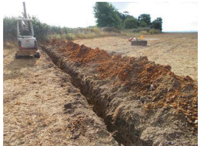
DP 12. Field south-west of the village. Cable trench, looking south-east.
