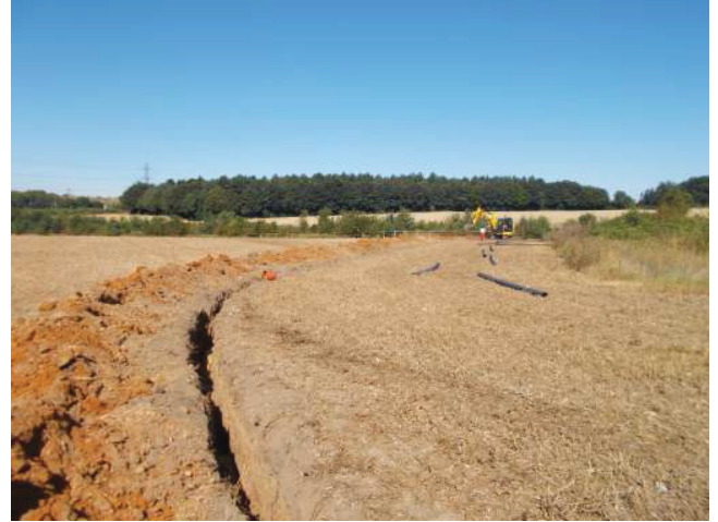
DP 14. Field south-west of the village. Looking north-west.
