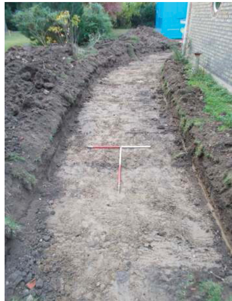
DP 22. Trench 6. Looking south.
