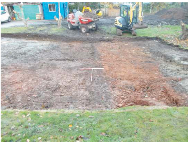
DP 5. Excavation area. Looking west-south-west.
