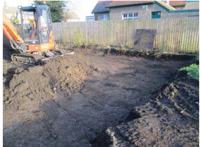
DP 2. Ground reduction undergoing. Looking north-north-east.
