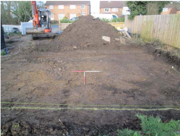
DP 3. Reduced ground area. Looking north-west.
