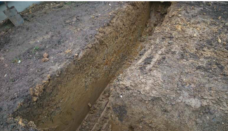
DP 10. South-west part of the trench. Looking west.
