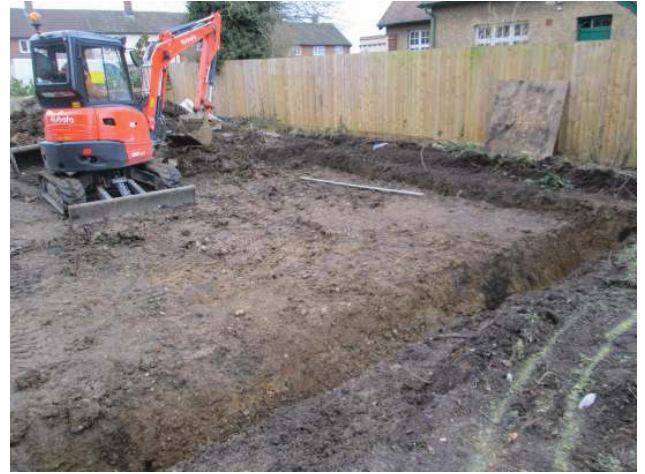
DP 8. Foundation trench. Looking north.
