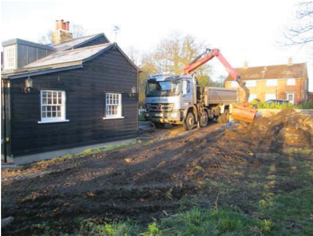
DP 1. The site. Looking west-north-west.
