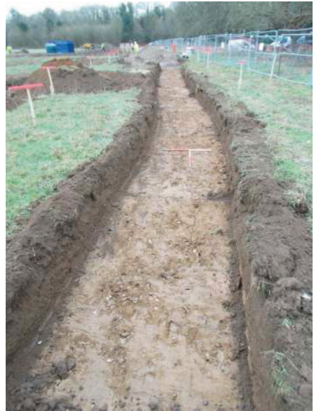
DP 2. Trench 1. Looking east-south-east.
