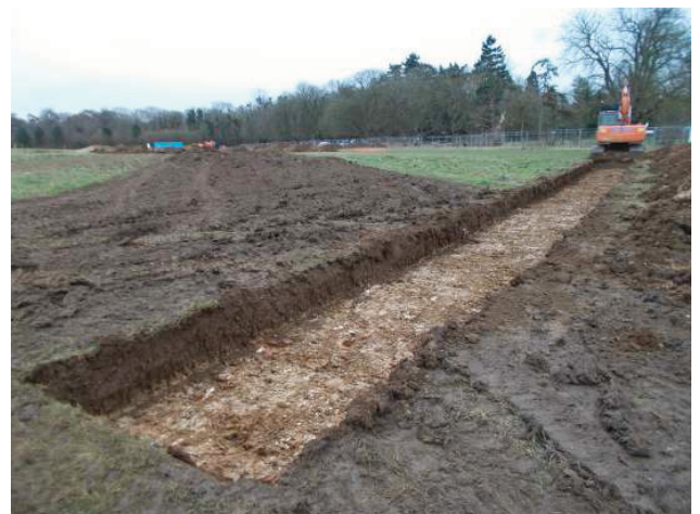
DP 12. Trench 4 before further excavation. Looking east-south-east.
