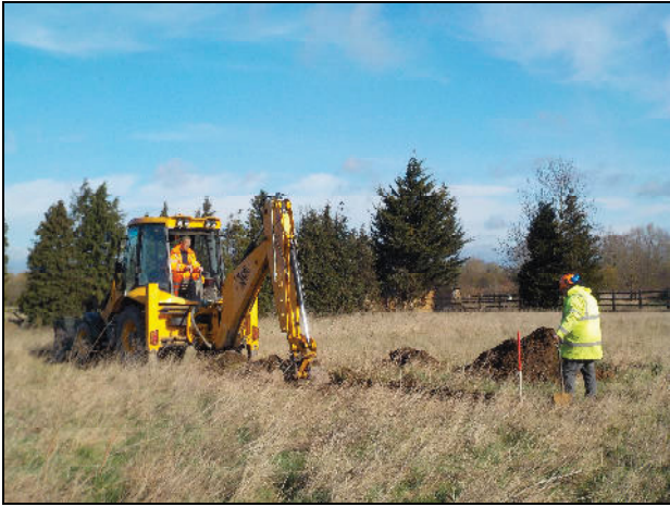
1 Trenches being excavated
