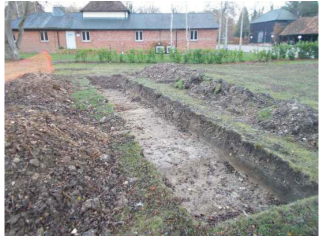
DP 44. Trench 8. Looking south.
