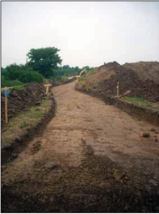
1 Haul road monitoring, June-July 2013
