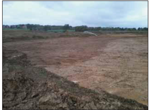
2 View of excavation area, February-March 2014
