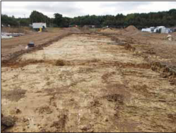
3 View of September 2016 excavation area Ci looking south
