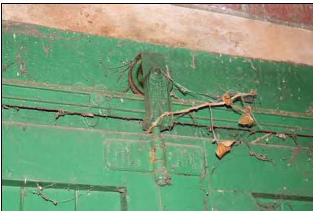
Detail of a hinge on a sliding door in Building 6 marked 'KING HITCHIN', taken from the north-east
