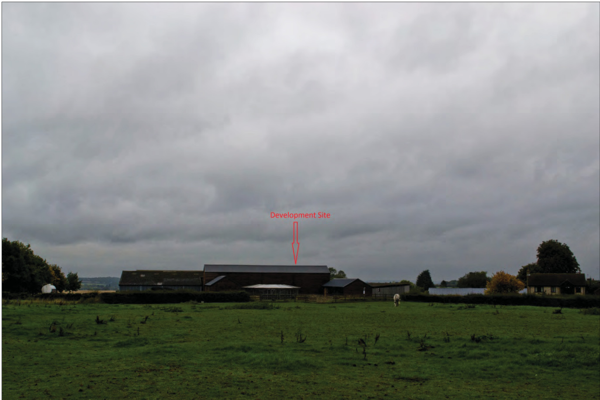
Plate 9. View towards development site from the footpath approaching 'The Hills' from the north
