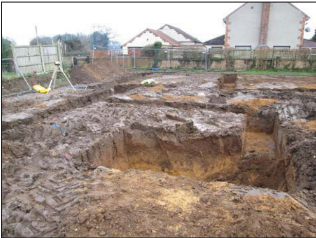
3 Complete footing excavation looking east
