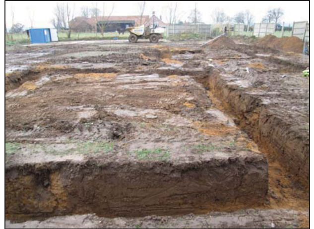
2 Complete footing excavation looking west
