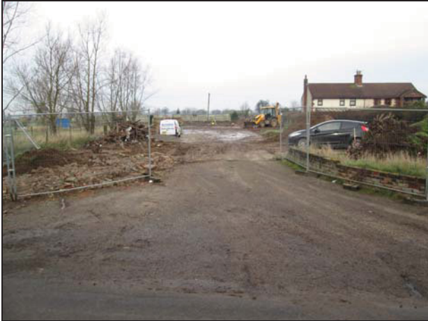
1 Entrance to the site looking north
