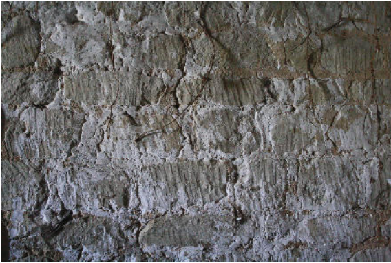
19: Example of tooling marks found on clunch stonework in Burwell
