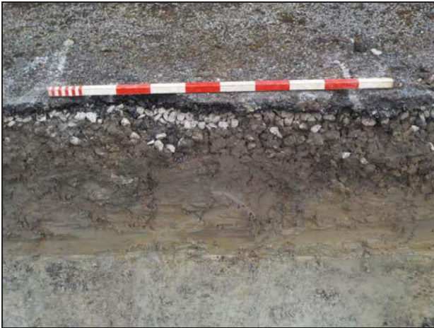
3 Sample Section 1A. Looking northwest.
