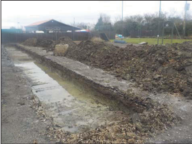
1 View of site. Looking northeast.
